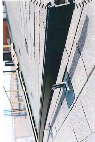
8. SEE RAIL ATTACHED TO L-FOOT.
