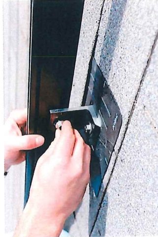
6. HAND TIGHTEN NUT UNTIL RAIL ALIGNMENT IS COMPLETE. VERIFY THAT POSITION INDICATOR ON BOLT IS VERTICAL (PERPENDICULAR TO RAFT).
