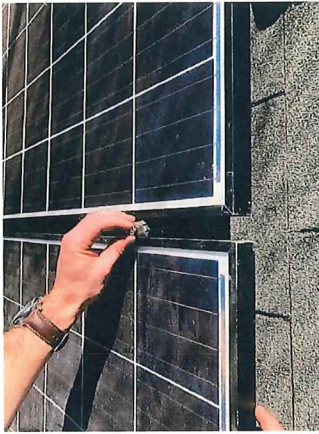
4. INSERT 1/4" T-BOLT INTO RAIL.
