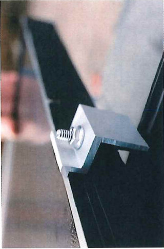
3. SEE MODULE ENGAGED BY ENDCLAMP.
