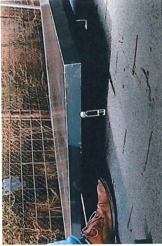
4. SEE MODULE ENGAGED BY ENDCLAMP.
