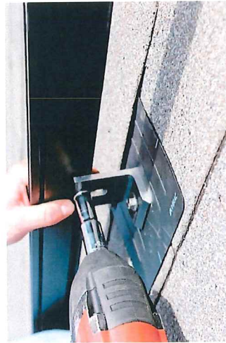
7. USE DRILL TO TIGHTEN NUT ONTO T-BOLT.
