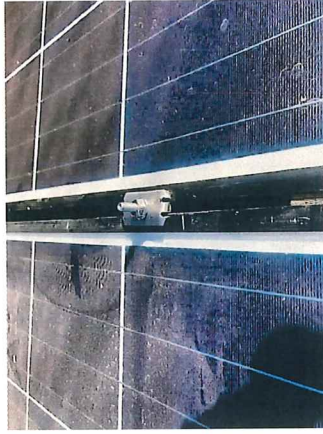
6. TIGHTEN NUT TO SECURE MODULES IN PLACE WITH MIDCLAMP.
