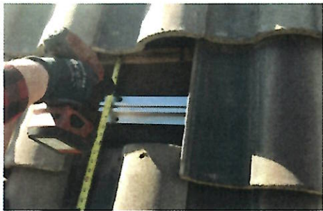
LOCATE RAFTER & DRILL PILOT Locate rafter where tile was removed and align tile replacement base mounting holes over rafter and vertically. Mark and drill pilot holes.
