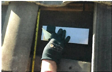
PREPARE UNDERLAYMENT & BUTYL Clear any pilot hole debris from underlayment and peel to remove sealing patch release liner.
