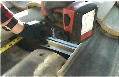
INSTALL BASE Optional: Place Tile Replacement Sub Flashing Align base over pilot holes and install base using supplied lag screws and sealing washers.
