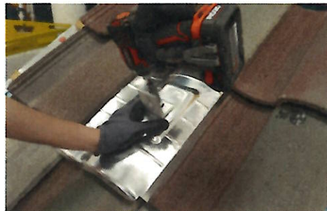
ATTACH L-FOOT: Install sealing L-Foot, Washer and Locknut. Fasten the nut on to the base of the L-Foot to 10 ft-lbs torque.
