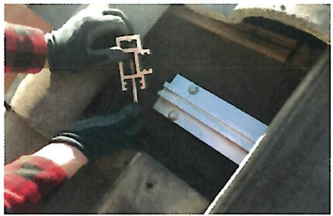
PREPARE RISER Assemble tile replacement riser and bolt using the correct configuration for tile type. (Can be completed before Base Installation; S-Tile Configuration Shown)
