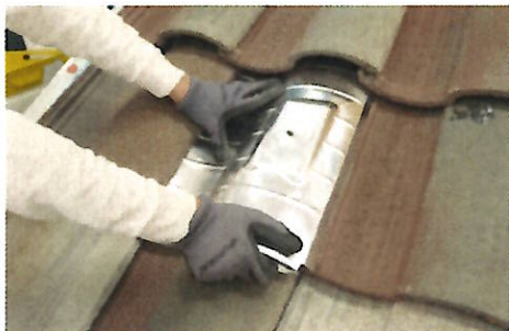
INSERT TILE FLASHING: Lift upslope and adjacent tile to insert tile flashing into tile course. Position replacement flashing over riser and insert into replacement flashing. Riser can be freely slid to position with mating flashing hole.
