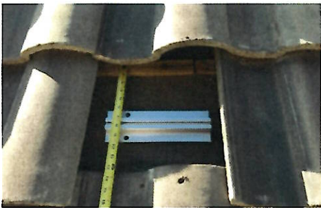
LAYOUT Locate rail attachment locations and remove corresponding tile that will be replaced by Unirac Tile Replacement.
