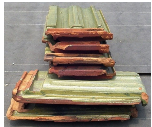
Side View - Staged Tiles (Slope ↓)
