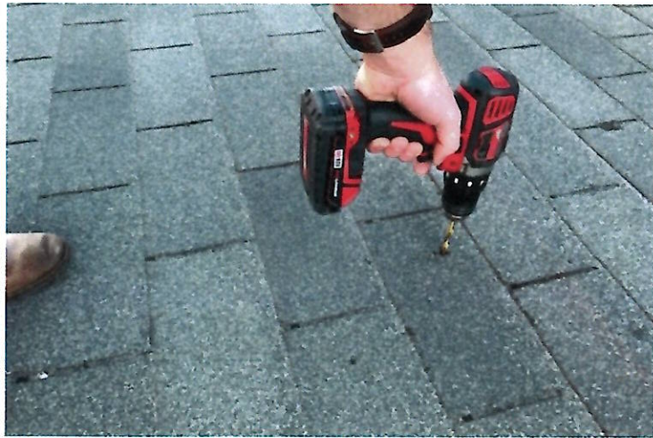
1. OVER THE RAFTER, DRILL A PILOT HOLE(S) FOR THE LAG BOLT(S).
