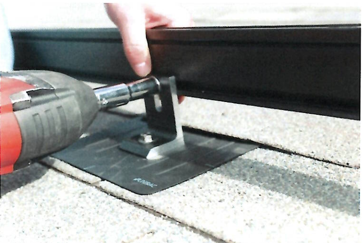
7. USE DRILL TO TIGHTEN NUT ONTO T-BOLT.
