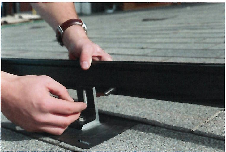
5. INSERT 3/8" T-BOLT INTO RAIL AT L-FOOT LOCATIONS. ROTATE T-BOLT INTO POSITION.
