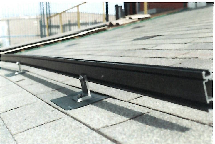
8. SEE RAIL ATTACHED TO L-FOOT.
