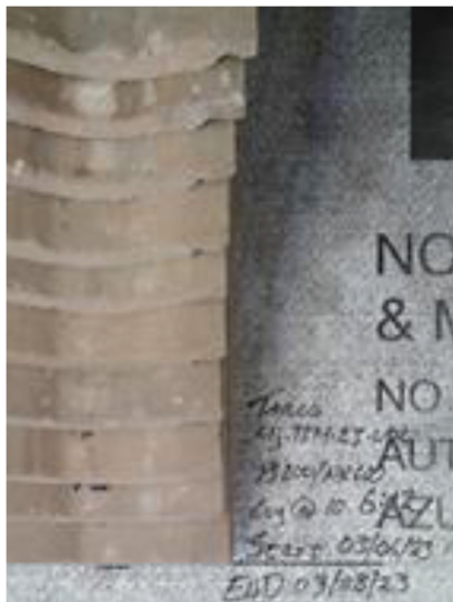
Side View - Staged Tiles (Slope ↓)
