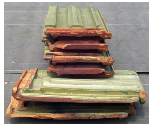
Side View - Staged Tiles (Slope ↓)
