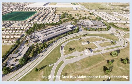
expense and reduce dead head miles. The bus facility entails bus operations, maintenance, parts storage, wash and service areas and employee/visitor parking. The site includes parking for one hundred (100) 60-foot articulated battery electric buses (BEBs) with charging capability. The Facility sits on a 20-acre site located near the southwest corner of the intersection of SW 127 Avenue and Biscayne Drive. The project delivery method has changed from Design-Build to Design-Bid-Build.
