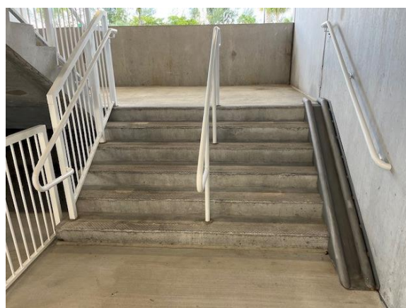
Figure 3- 22: Existing Bicycle Ramp at the Golden Glades Multimodal Transportation Facility
