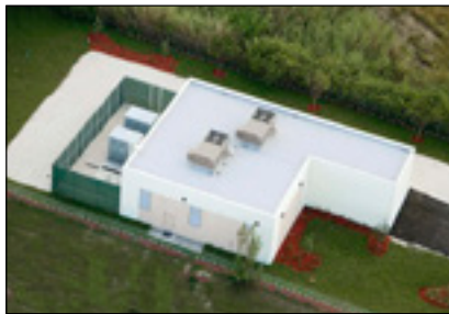
Palmetto Traction Power Sub-Station
