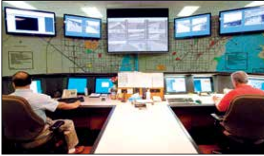
Traffic Control Center
