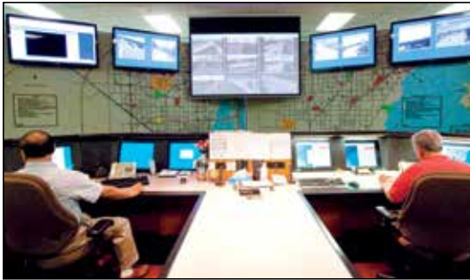
Traffic Control Center
