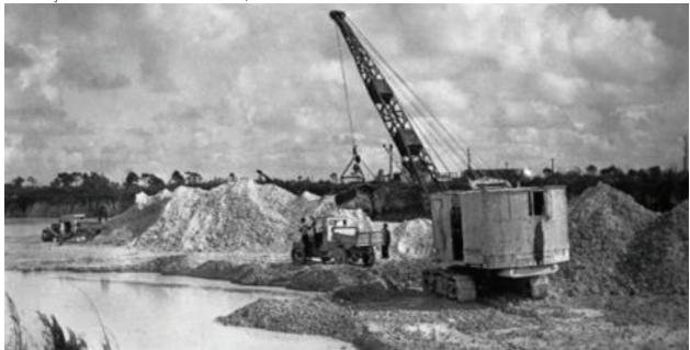
Figure 13: FERA mining rock for road construction in Dade County in 1935 (Florida Memory)
