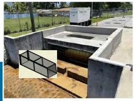
Installed in Discharge Alt of Energy Dissipater Only One Section Shown of Two Part Assembly
