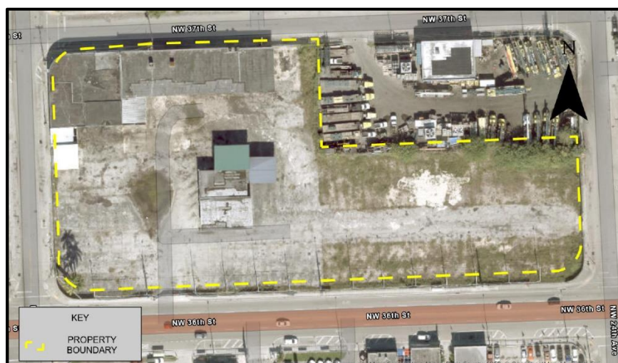
Bindi Investments Site pre-redevelopment
