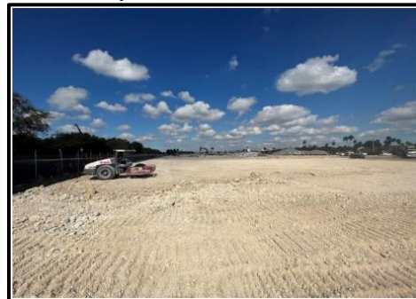
Site cleared for redevelopment
