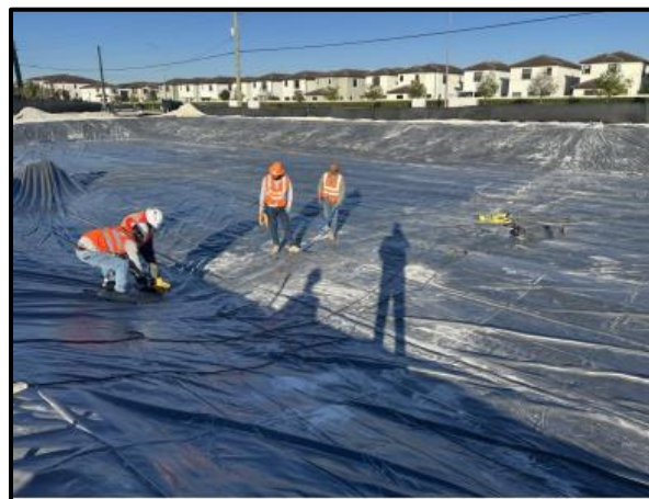
Liner installed in retention area
