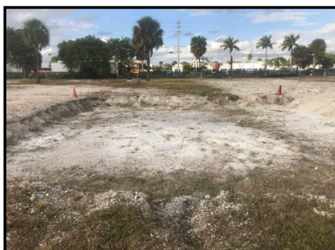
Excavation at the site
