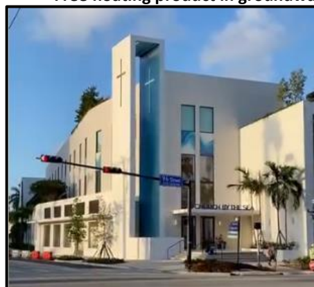
Completed Church By the Sea
