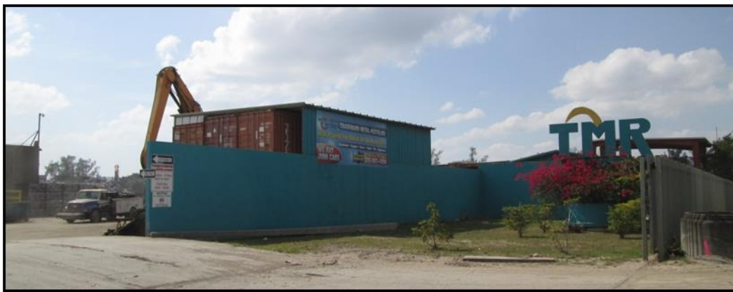
Trademark Metals Recycling Facility
