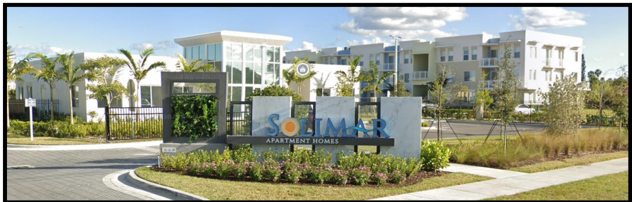
Completed Solimar Apartments
