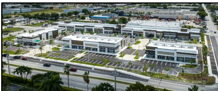
Completed Doral 87 Brownfield Site
