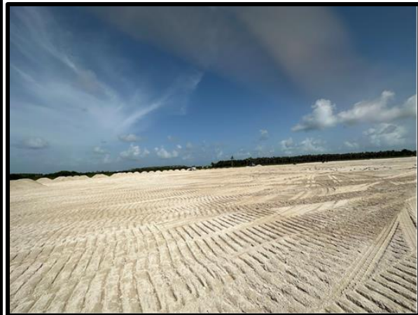
Clean fill engineering control installed
