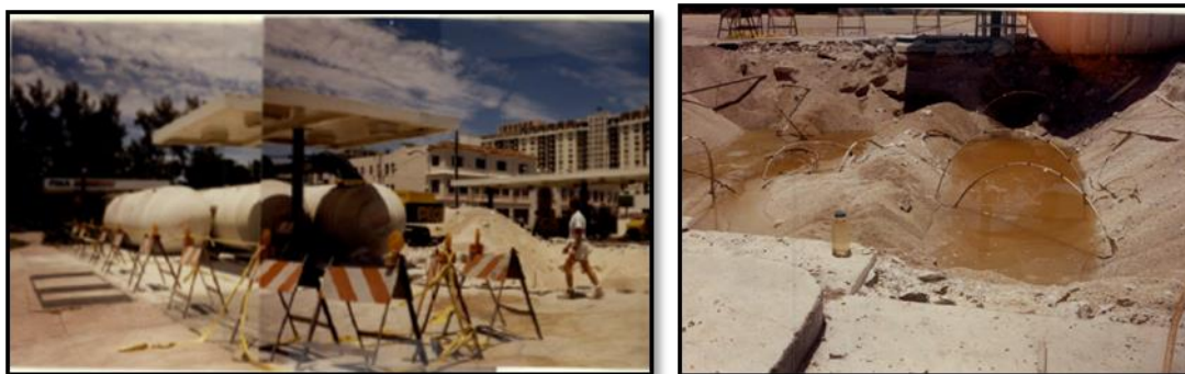
Historic underground storage tank removal (1991)
