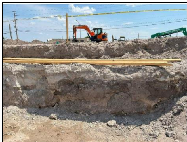
Soil profile during foundation construction
