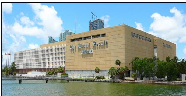
Former Miami Herald Building
