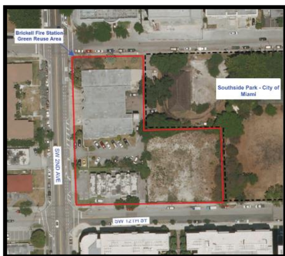
Brickell Fire Station Site prior to redevelopment
