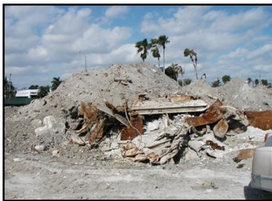
Solid Waste excavated
