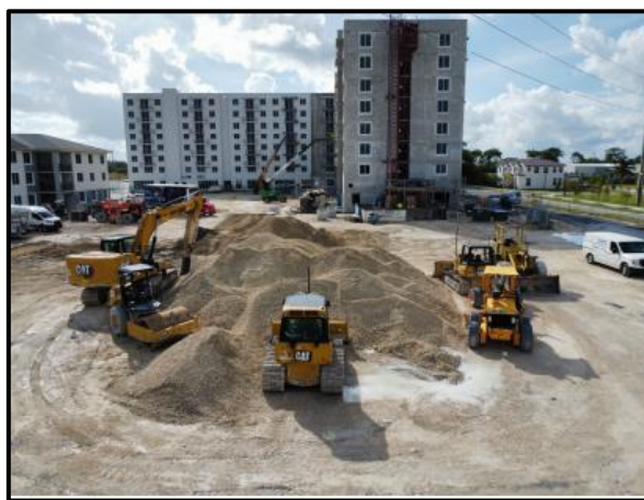
Soil management activities occurring December 2024
