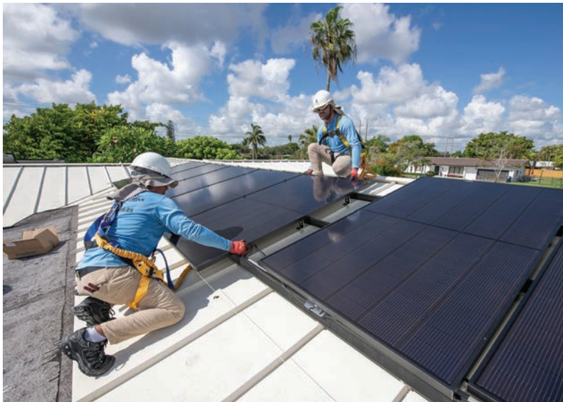
Solar panels are installed on a solar co-op members home.
