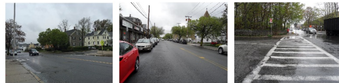
Allston Street Curb Extension
