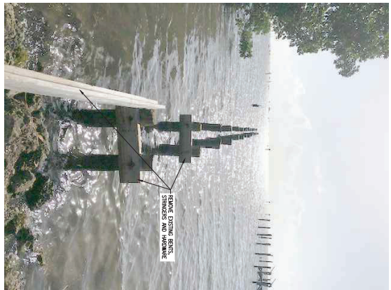
PHOTO SD101-3 EXISTING DOCK PILES
