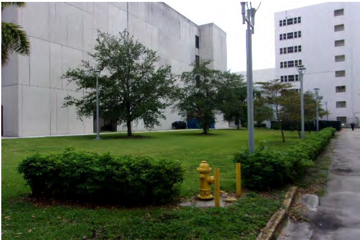
LOOKING NORTHEASTERLY AT SUBJECT
