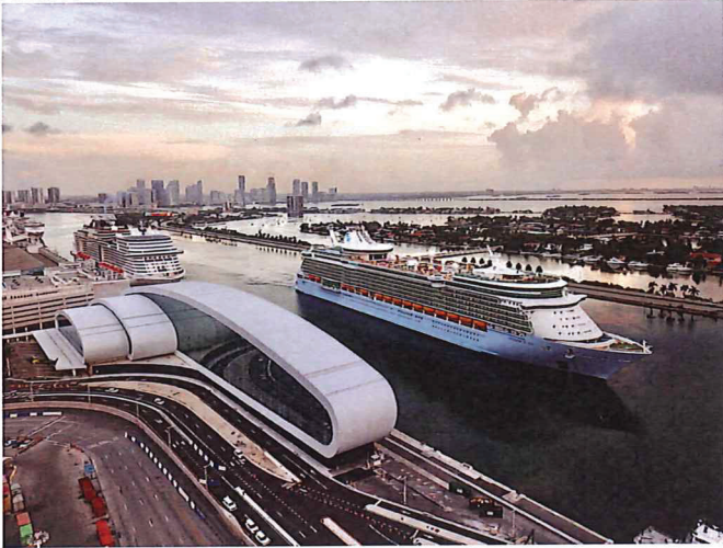
Figure 2: Photograph of Cruise Terminal B at PortMiami, which received LEED Gold certification in November 2021.
