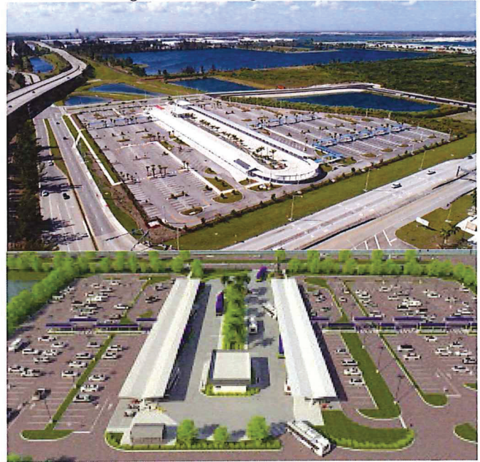
Figure 3: Photographs of Miami-Dade County's first two infrastructure projects to use the Envision rating system. The Dolphin Station Park and Ride (top) and Tamiami Station Park and Ride (bottom) utilized sustainable design and construction practices that included increasing permeable surface area and coordinated integration to existing transit infrastructure.
