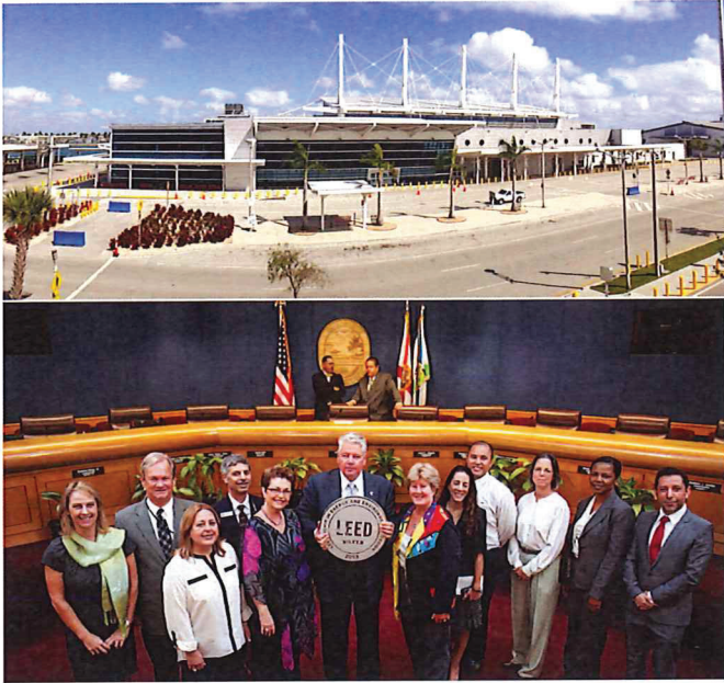
Figure 4: Photographs of renovations and new construction at the Port of Miami Terminal D (top). The Port has successfully completed a number of sustainable building projects that include HVAC system upgrades, low-flow water uses plumbing fixtures, cool roofs, and more. Terminal D received LEED Silver certification in September 2013 (bottom).
