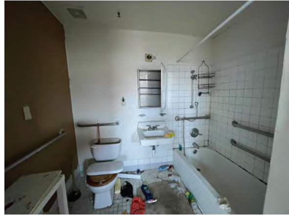
Photo 14 – Typical ADA Bathroom
