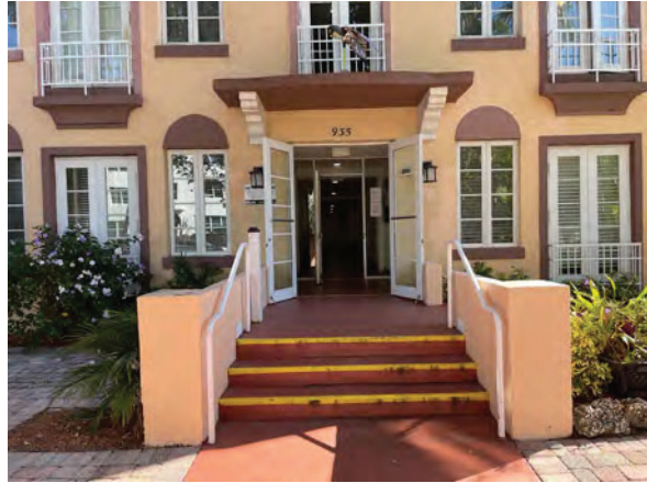
Photo 2 – Front Elevation & Approach
