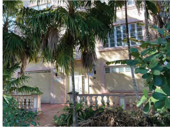
Photo 2 – Front Elevation & Approach
