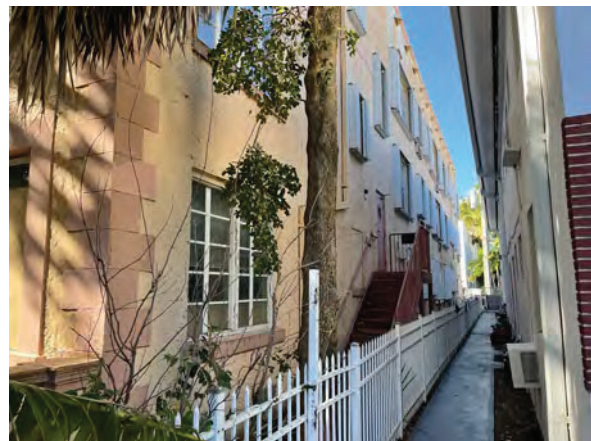
Photo 18 – North Side Elevation
