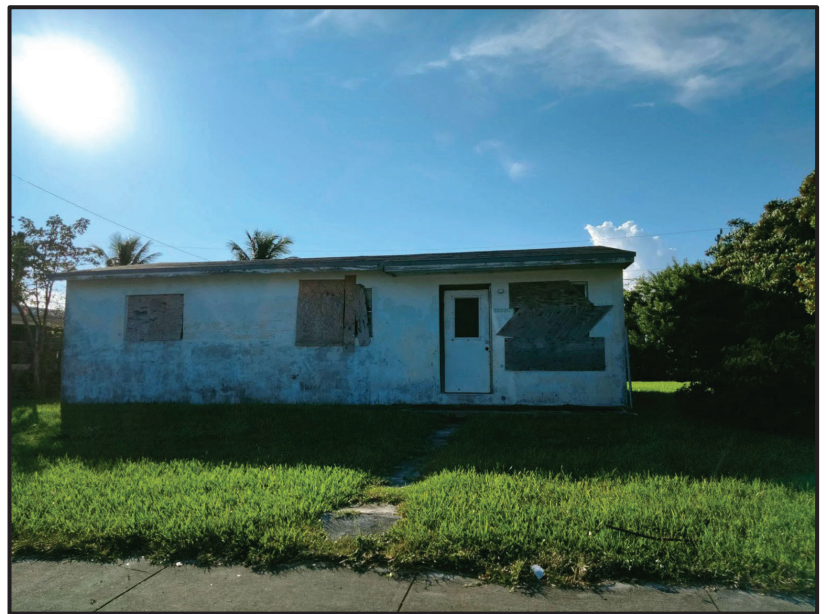
Photo credit: Stuart Architecture, 01/24/22
