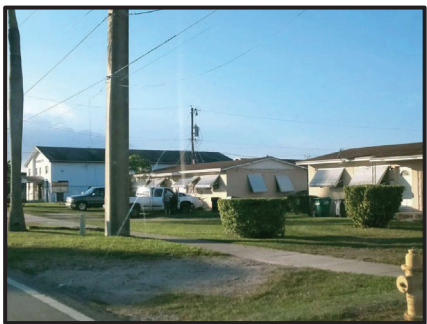
Photo credit: Stuart Architecture, 01/24/22
