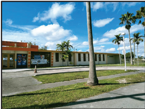
Photo credit: Stuart Architecture, 01/17/22
