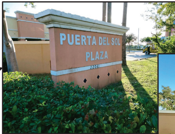
Photo credit: Stuart Architecture, 01/24/22
