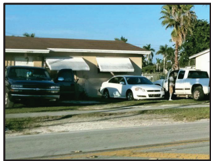
Photo credit: Stuart Architecture, 01/24/22
