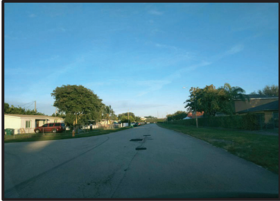
Photo credit: Stuart Architecture, 01/24/22
