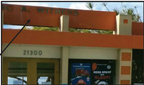
Photo credit: Stuart Architecture, 01/17/22
