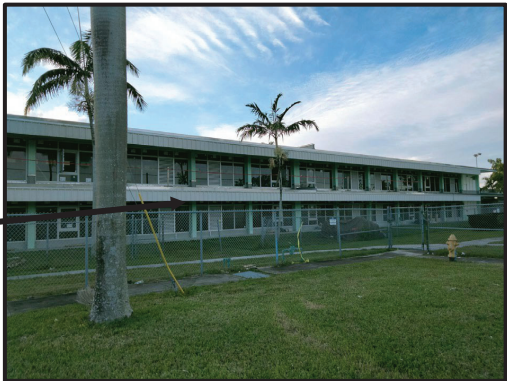
Photo credit: Stuart Architecture, 01/24/22
