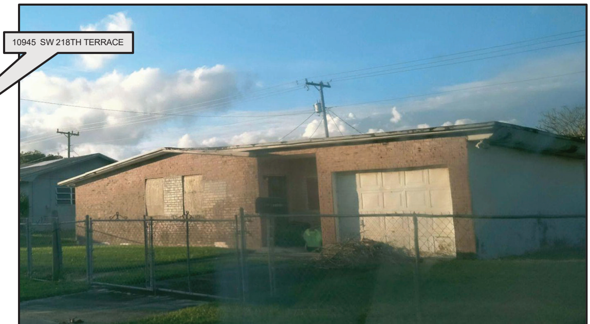
Photo credit: Stuart Architecture, 01/24/22
