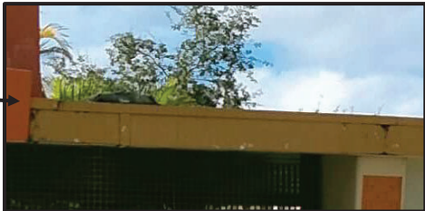
Photo credit: Stuart Architecture, 01/17/22
