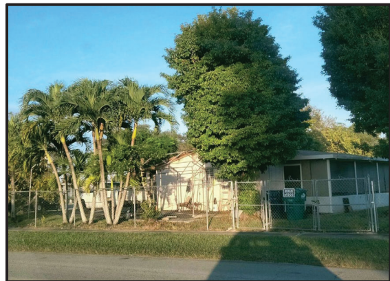
Photo credit: Stuart Architecture, 01/24/22
