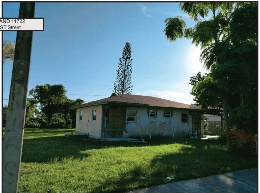
Photo credit: Stuart Architecture, 01/24/22
