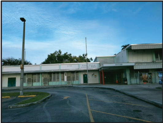
Photo credit: Stuart Architecture, 01/24/22
