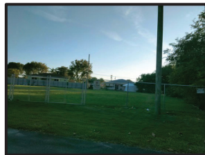
Photo credit: Stuart Architecture, 01/24/22
