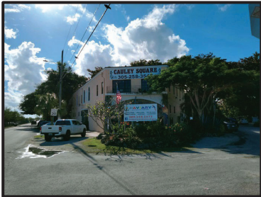
Photo credit: Stuart Architecture, 01/17/22
