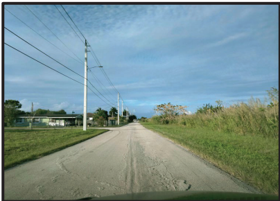
Photo credit: Stuart Architecture, 01/24/22
