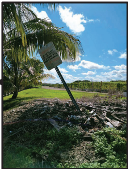
Photo credit: Stuart Architecture, 01/17/22
