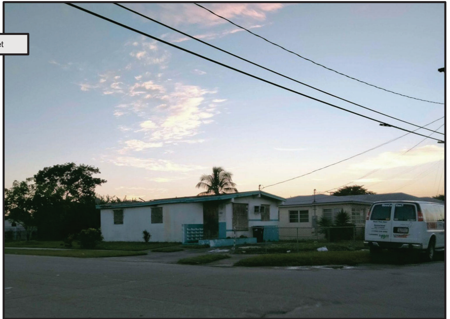
Photo credit: Stuart Architecture, 01/24/22
