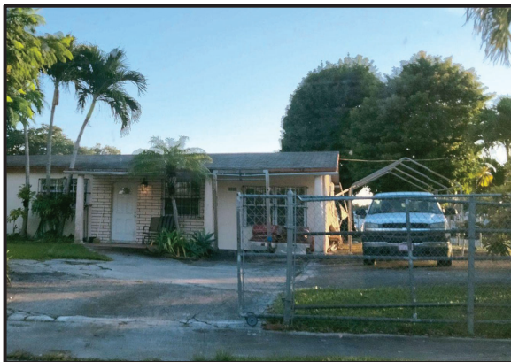
Photo credit: Stuart Architecture, 01/24/22
