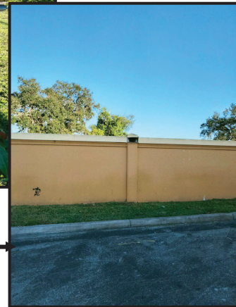
Photo credit: Stuart Architecture, 01/24/22
