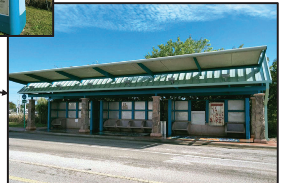
Photo credit: Stuart Architecture, 01/17/22
