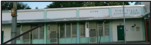
Photo credit: Stuart Architecture, 01/24/22
