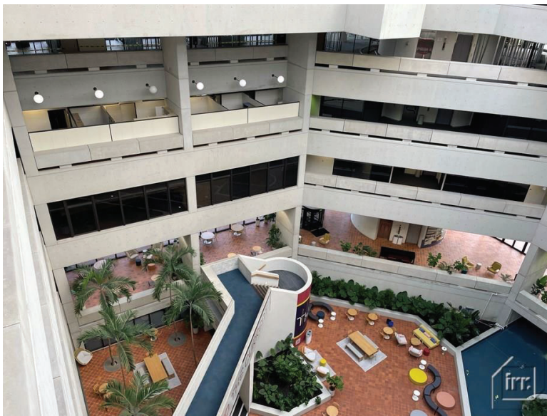
The Current (former FPL Operations Center) 9250 W. Flagler St. Miami, Florida
