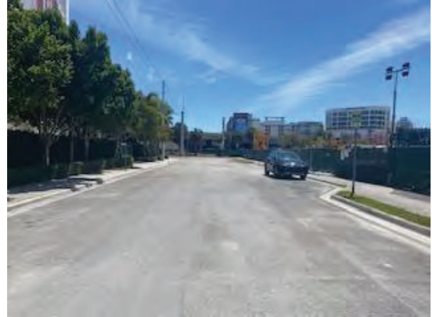
NW 9 th Avenue looking south (subject to right of photograph)
