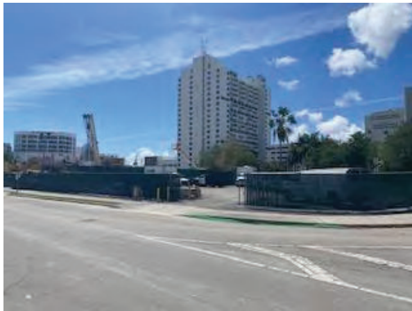
View of subject Folio Nos. 01-3135-019-2700 and 01-3135-019-2690 looking southwest from NW 9 th Avenue
