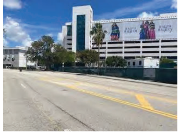
View of subject Folio Nos. 01-3135-019-2700 and 01-3135-019-2690 looking northeast from NW 10 th Avenue
