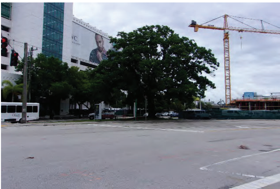
LOOKING SOUTHEASTERLY AT PARCEL 1 FROM N. W. 10 TH AVENUE
