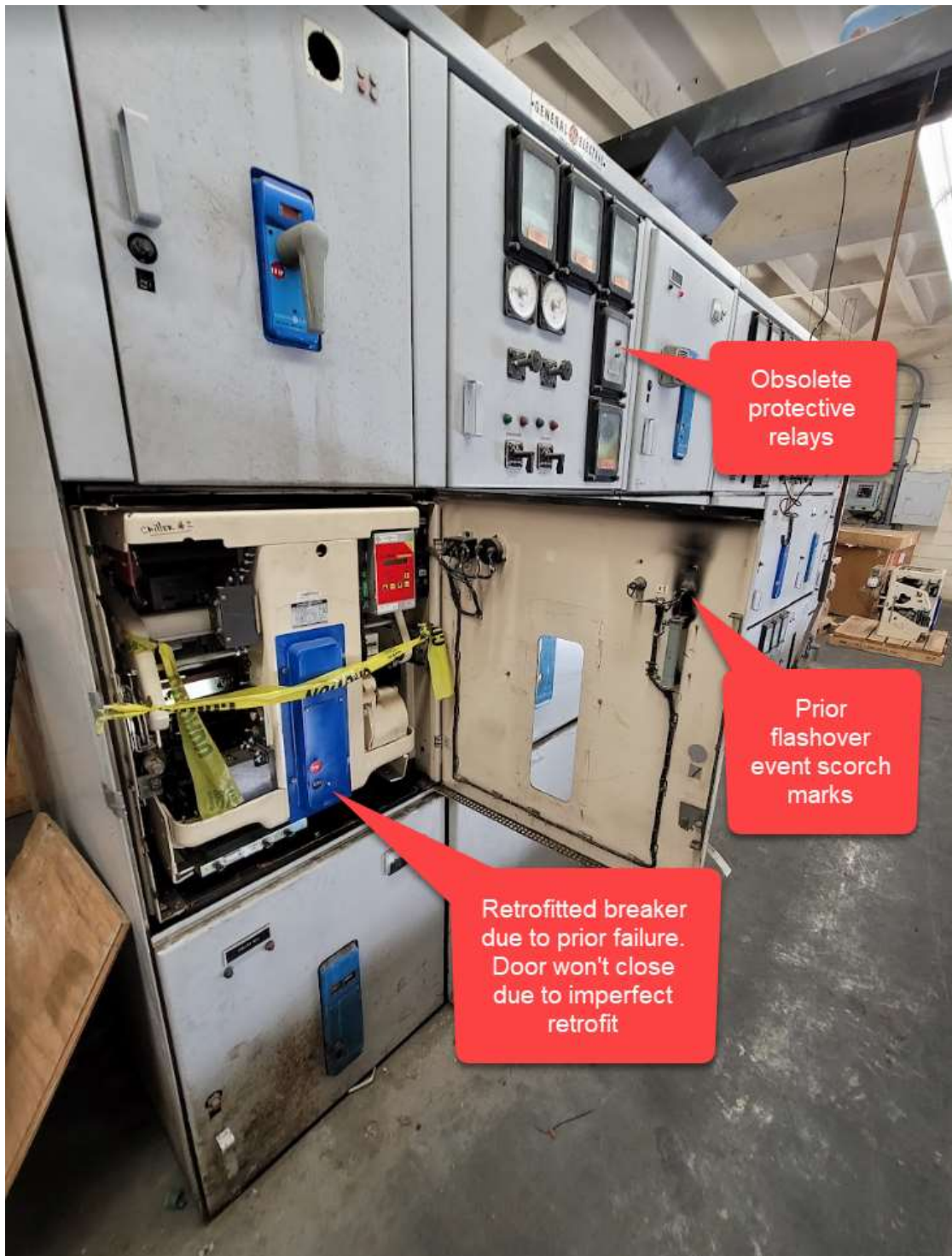
Figure 4 - Safety Issue with retrofitted breaker
