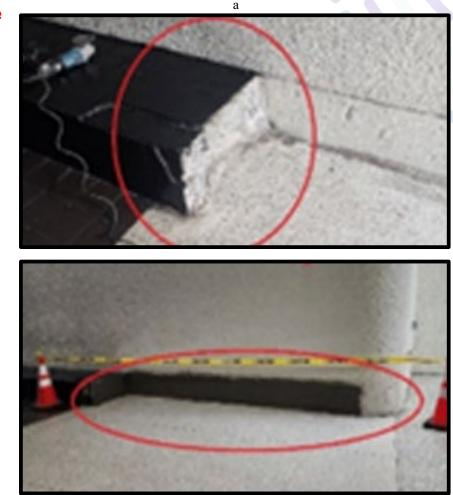
This project entailed the cutting, squaring and patching of a stationary tiled bench outside Door No. 12. Additional work entailed ensuring the bench was flushed and sprayed to blend in with the existing wall. The repair improves vision and contributes to a safer environment. The task was completed on January 27, 2025.
