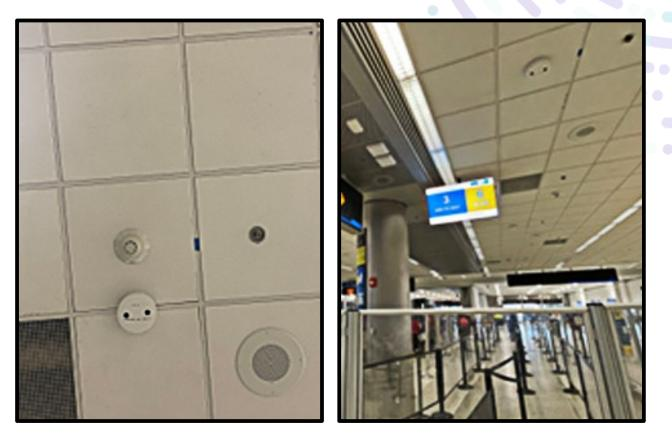
This project installed 3D sensors at Security Checkpoint 3. These sensors utilize advanced algorithms for queue management, real-time tracking and predictive modeling. The data collected from these sensors is stored enabling MIA officials to make well informed and real-time decisions regarding the effective management of checkpoint flows.
