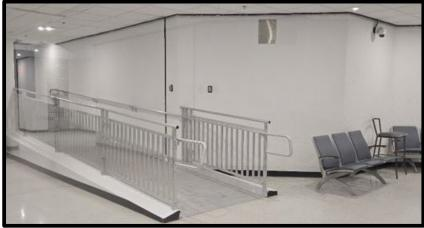
A prefabricated ADA accessible ramp was installed in the existing domestic bus lobby area at the ramp level. The new ramp offers access between the elevator vestibule and the bus lobby area. This project began in October 2024 and was completed in March of 2025.
