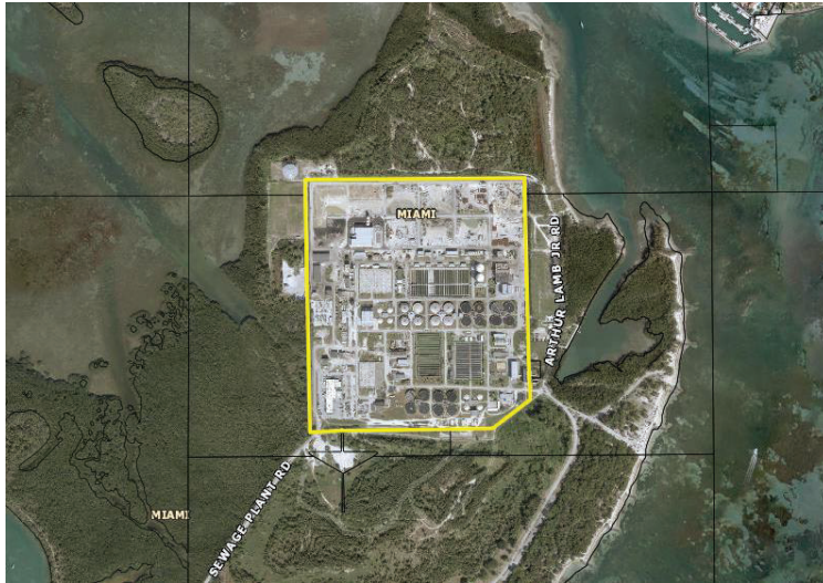
Central District WWTP (Courtesy MDPA)
