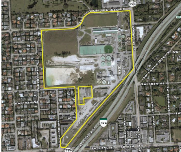
Alexander Orr WTP (Courtesy MDPA)
