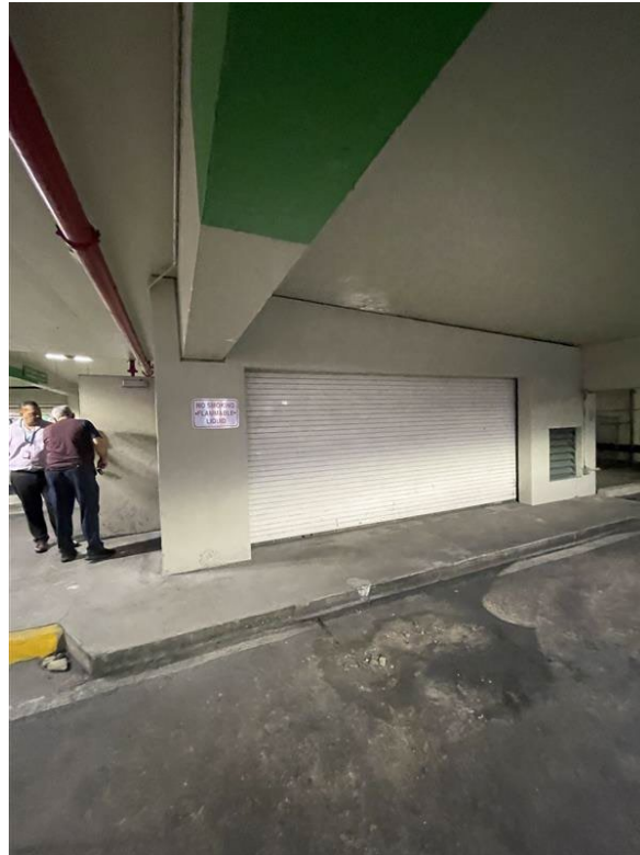
Figure 4.16 – Space outside room hosting diesel tank
