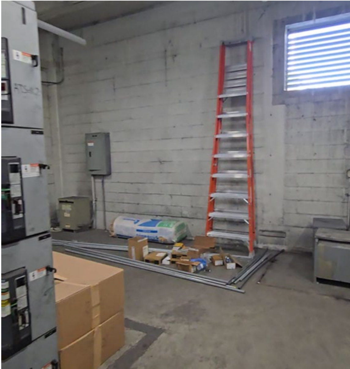
Figure 5.15 – Exterior (west) wall of switchgear room. Switchgear #2 to left of photo.
