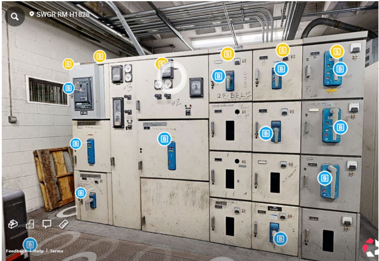
Figure 3.11 – Matterport image of MDS#2. Main exterior door to room to left of image. Loads include some H gates.
