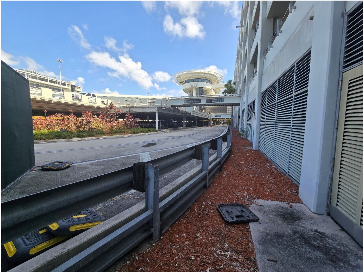
Figure 5.17 – Road/shoulder outside of electrical and switchgear rooms. Potential landing area for temporary equipment and general construction access. Photo faces north from switchgear room doors.
