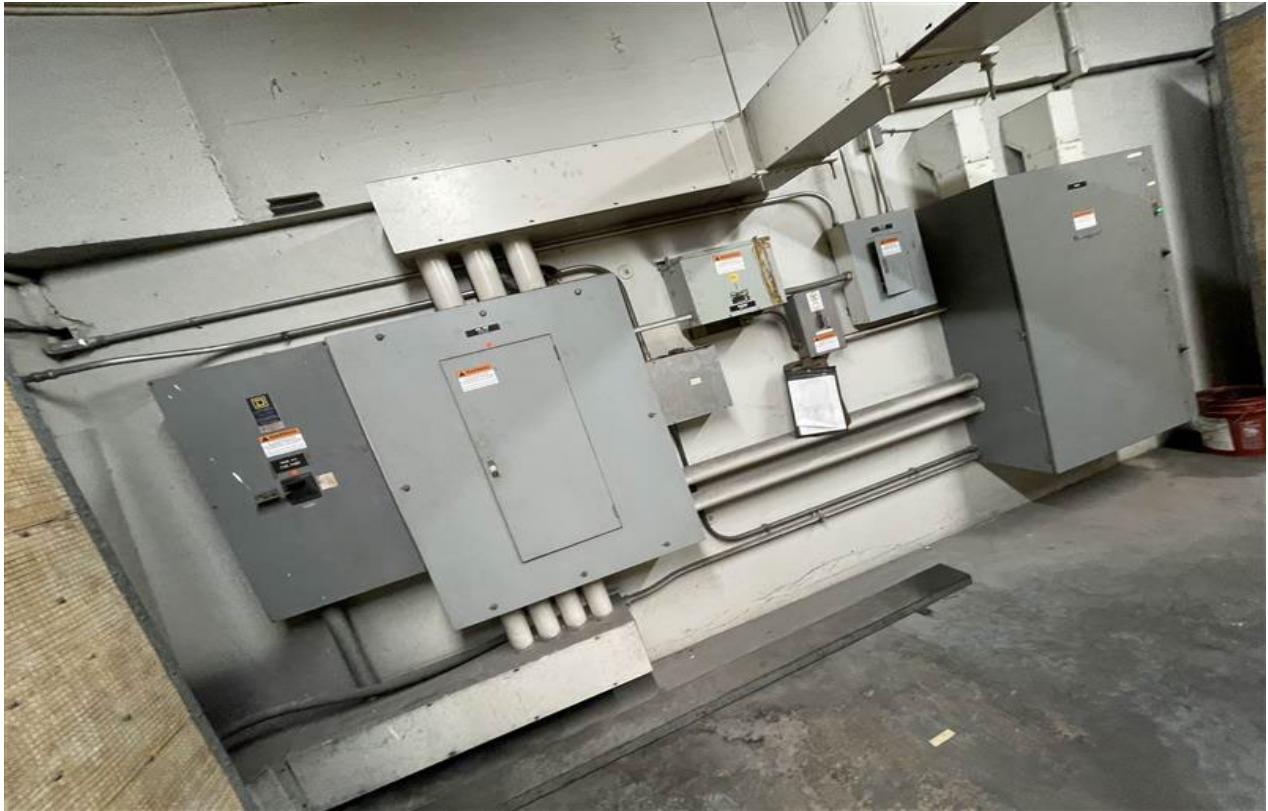
Figure 4.6 – North wall of generator room
