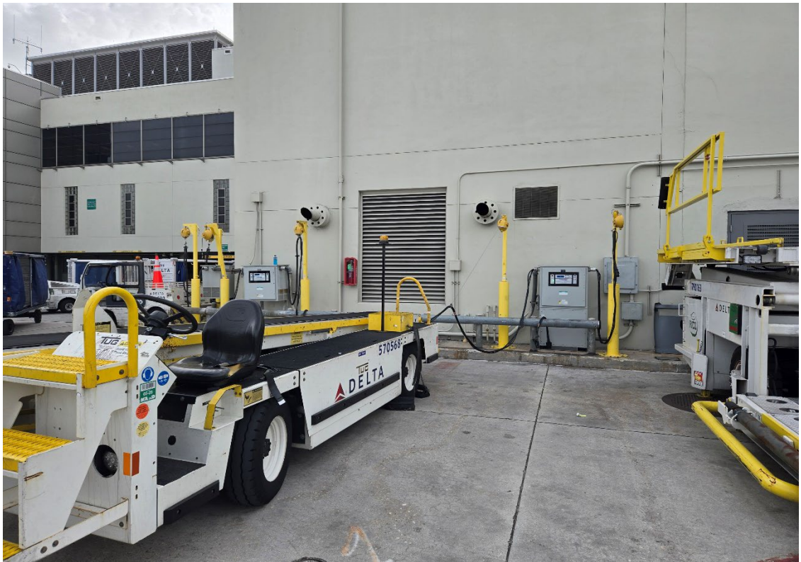
Figure 3.2 – Existing space outside of generator and electrical rooms.
