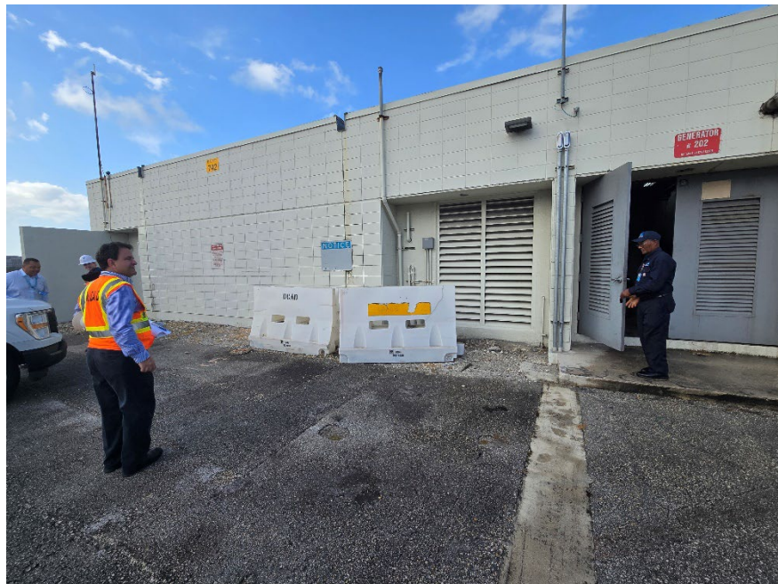
Figure 1.11 – Outdoor area in front of Bldg. 742
