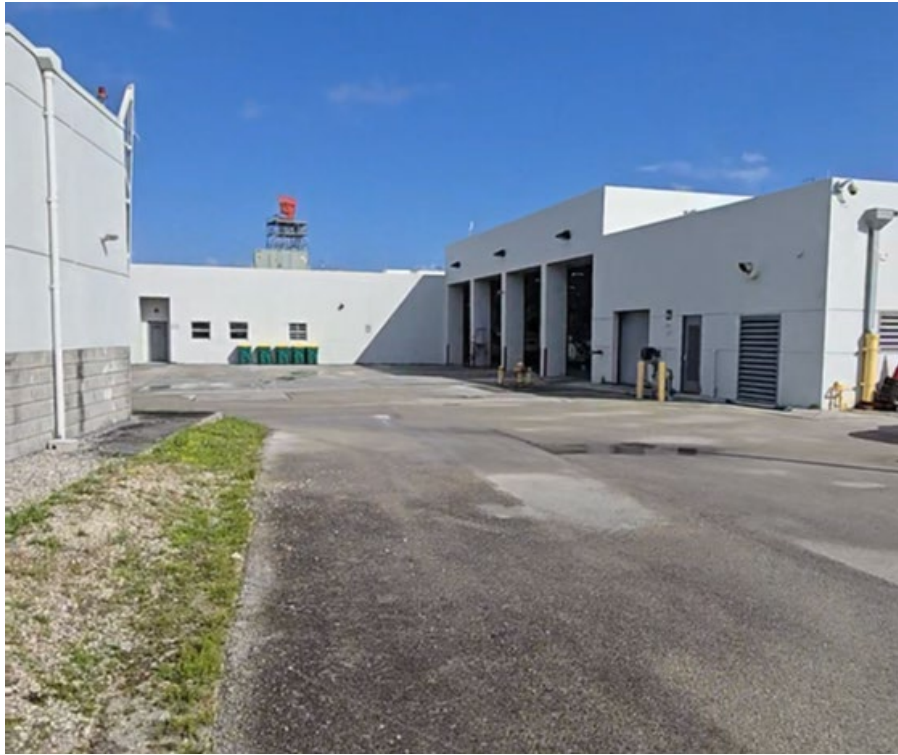
Figure 2.21 – Open paved area on north side of building, facing west
