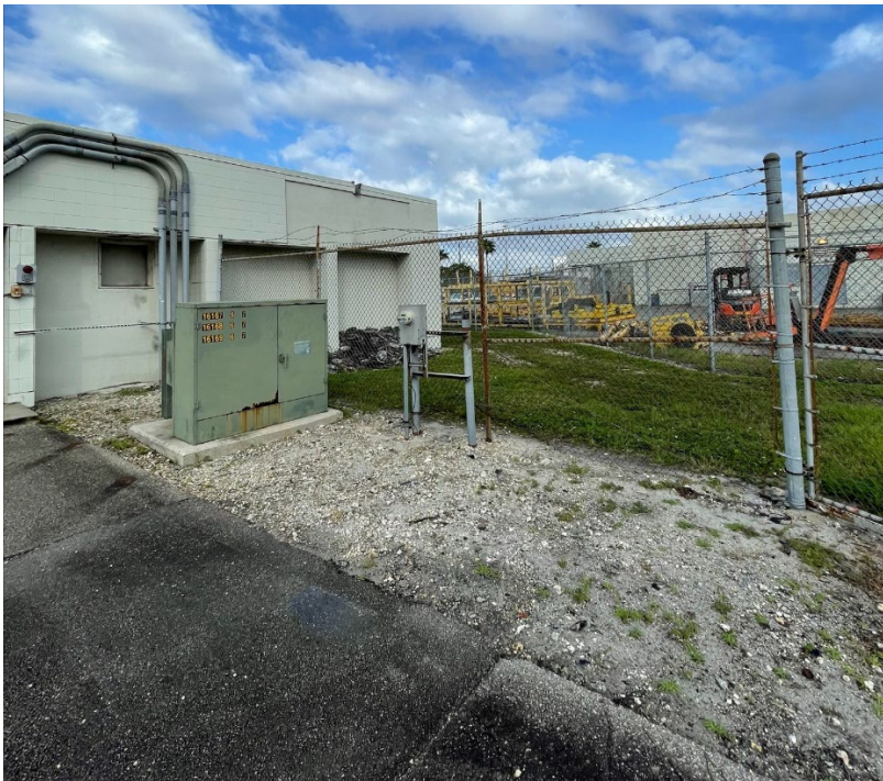
Figure 1.13 – Outdoor area in front of Bldg. 742
