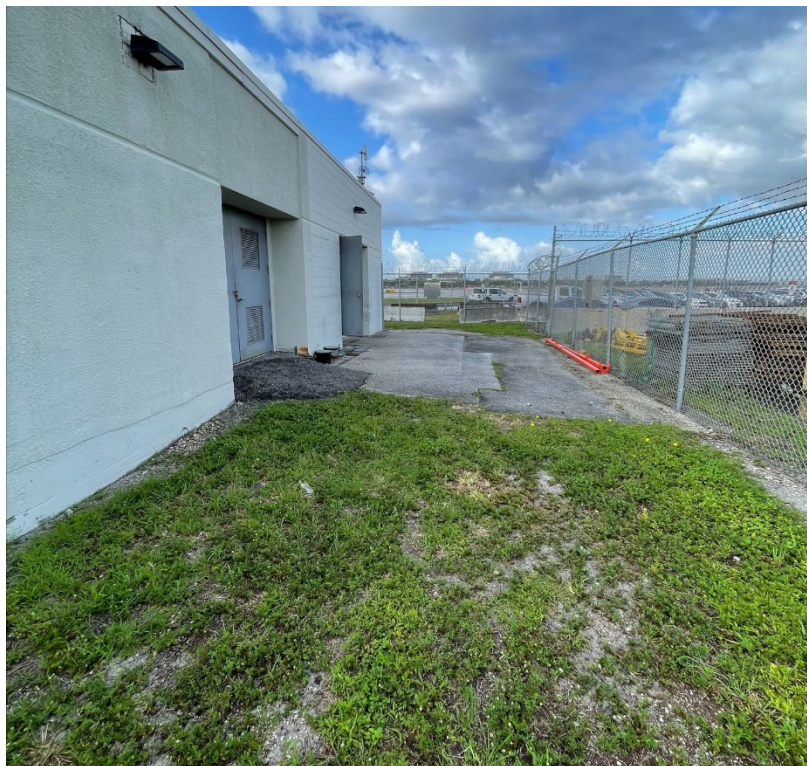
Figure 1.9 – Area outside lighting room entry doors to potentially house temporary equipment.
