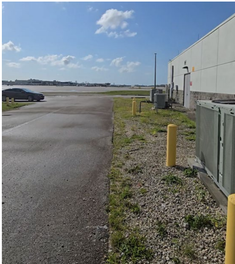
Figure 2.20 – Open paved area on north side of building, facing east
