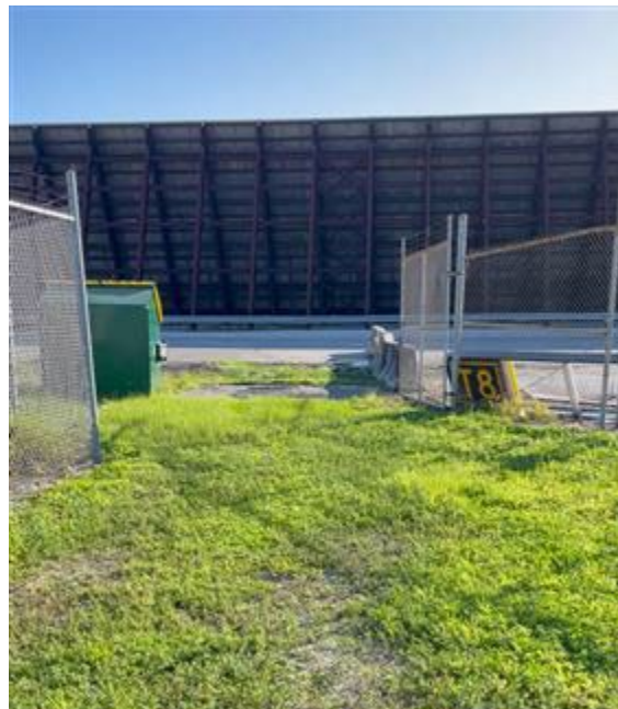
Figure 1.15– Grassy area leading to west side of the building
