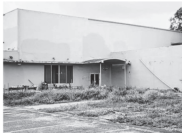
The Old Dillard Museum's 'Sistrunk Then & Now' exhibit shows photos of the Fort Lauderdale neighborhood through the years, including landmarks, night clubs and residential areas. This photo shows the vacant building that eventually would replace the old Elks Lodge.
