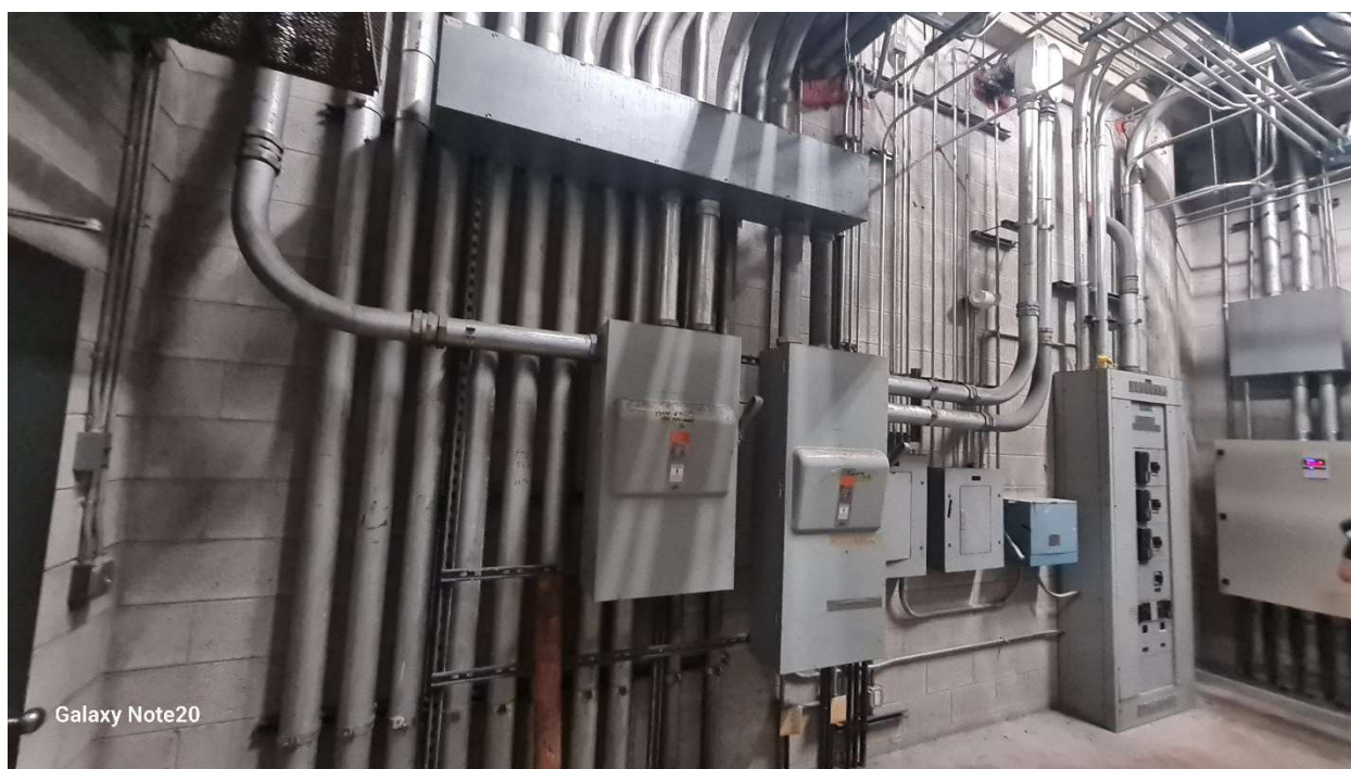
Figure 5.15 – South wall of switchgear room – wide angle
