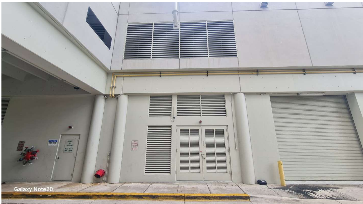
Figure 5.19 – Exterior frontal view of generator room (2 nd floor) and FPL vault (1 st floor).
