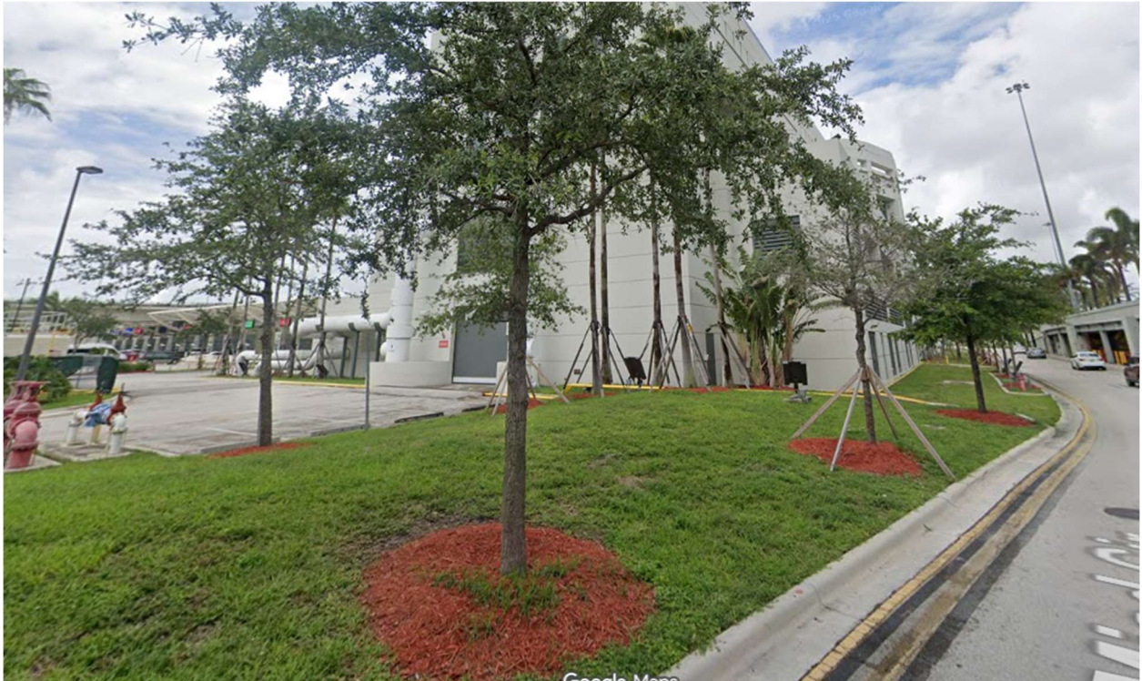
Figure 3.13 – Google Earth view of parking area on west side of Chiller Building
