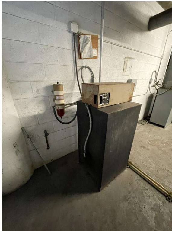
Figure 5.9 – Side view of diesel day tank
