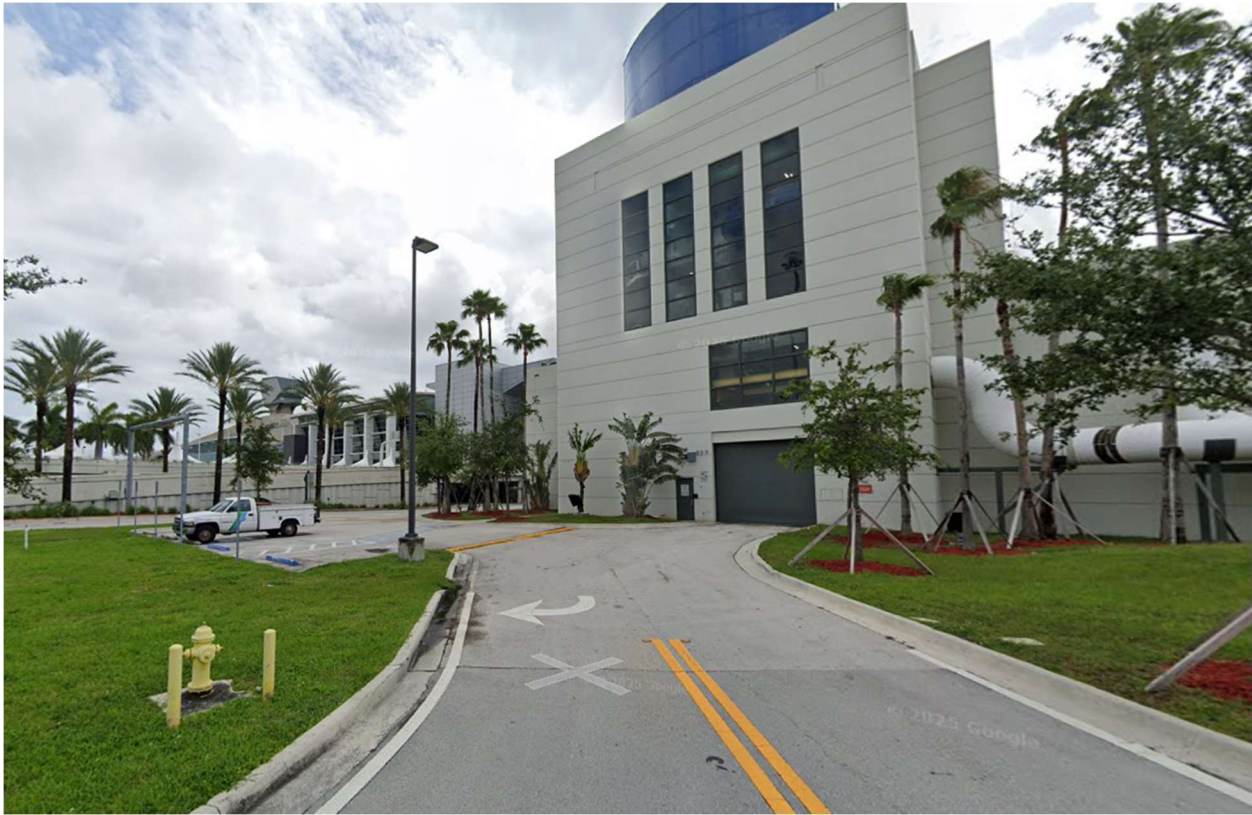
Figure 3.14 – Google Earth view of parking area on east side of Chiller Building
