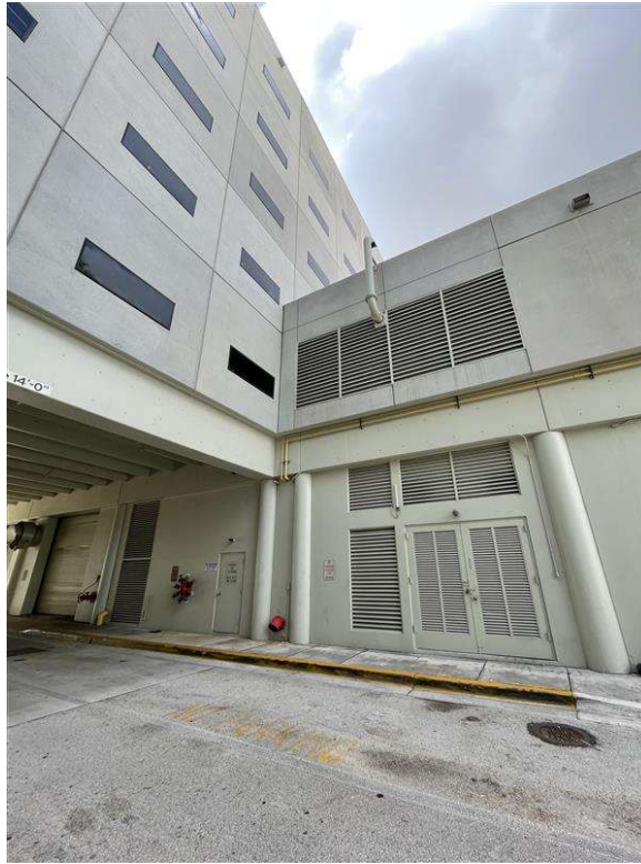
Figure 5.18 – Exterior view of generator room (2 nd floor) and FPL vault (1 st floor). Chiller room entrance to left in photo.
