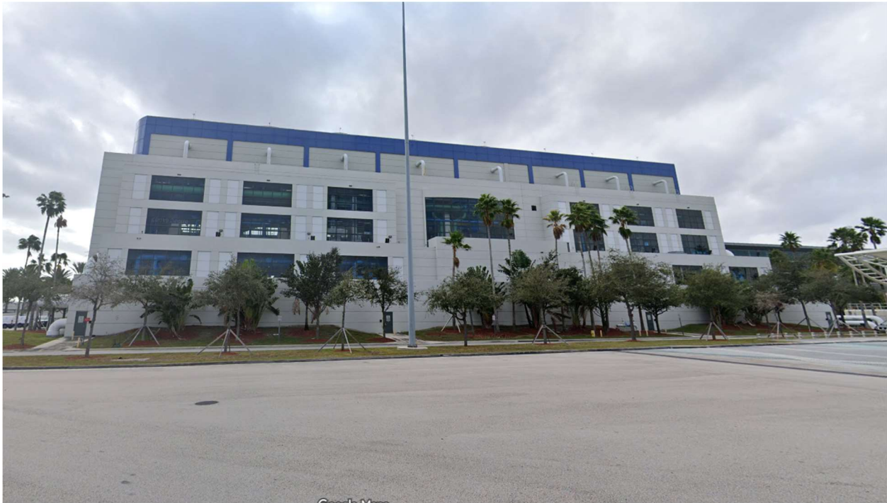
Figure 3.15 – South view of Chiller Plant, taken from toll plaza.
