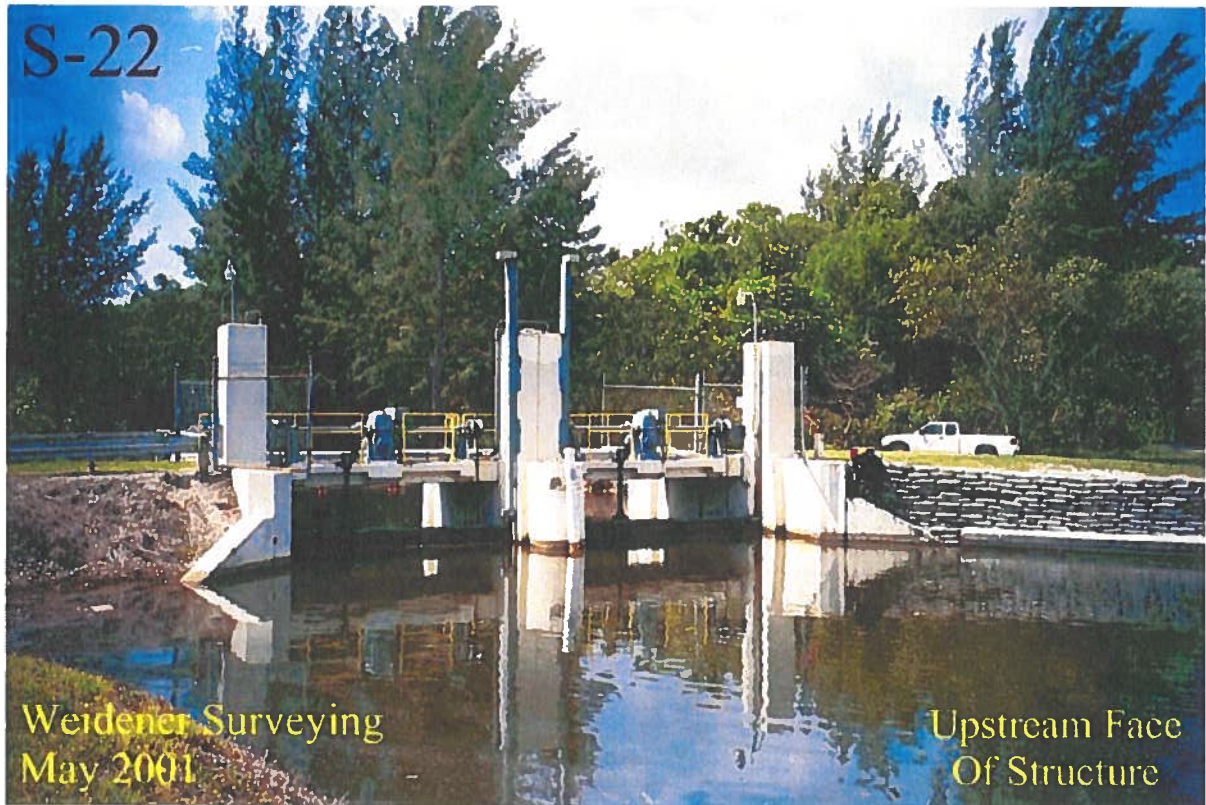
Figure 2: Structure S-22 - Upstream View
