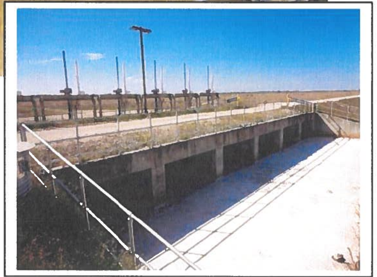
Figure 2: External View of Structure G-423: (top) Headwater, (bottom) Tailwater
