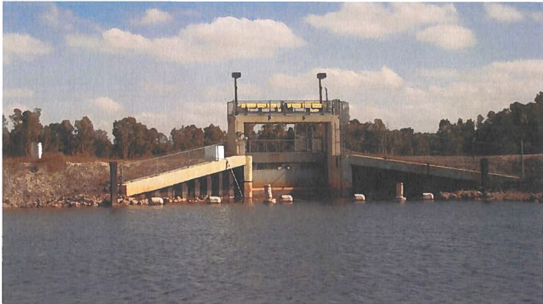
Figure 2: Structure G-421 – External View (Looking East)
