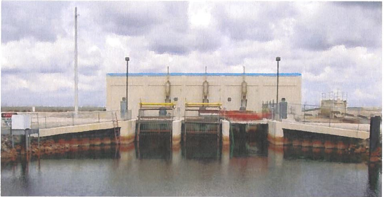
Figure 3: G-420 Pump Station – Looking west
