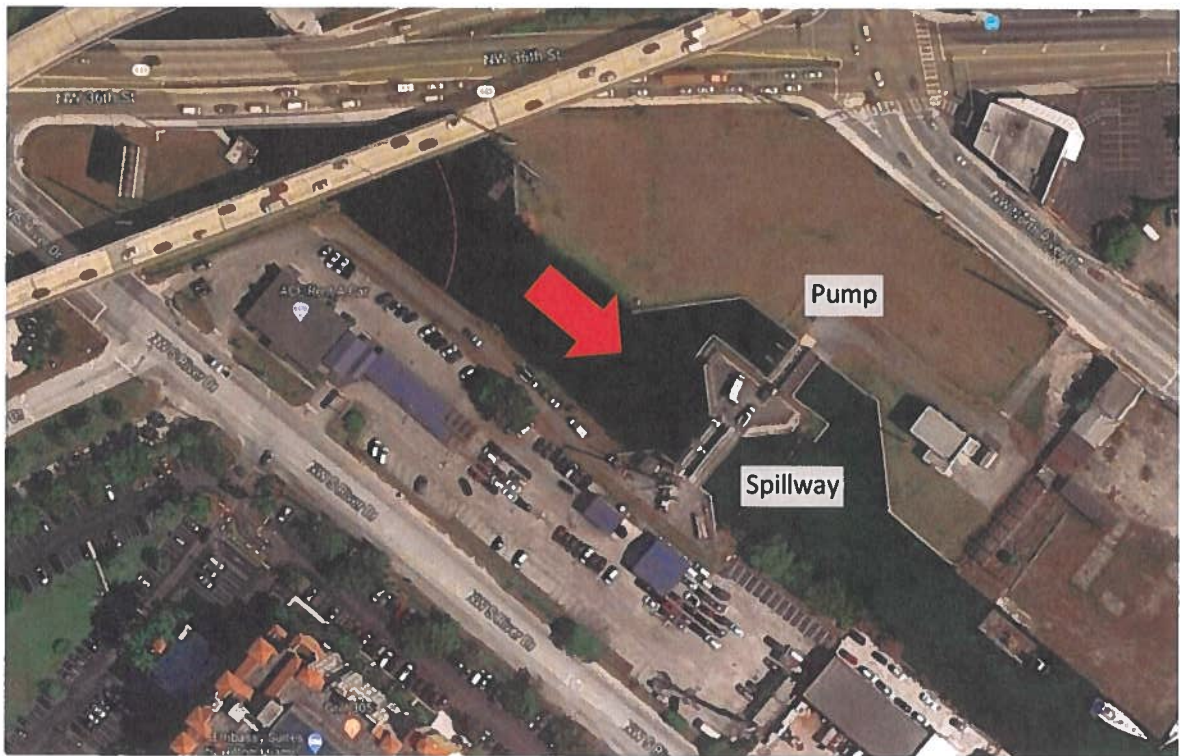
Figure 2: Structure S-26 Aerial View
