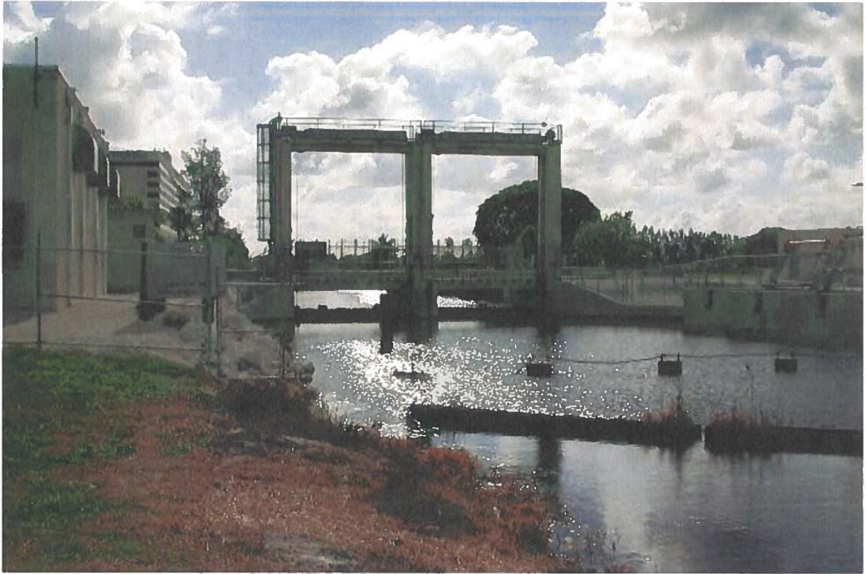
Figure 2: Structure S-25B- Upstream View
