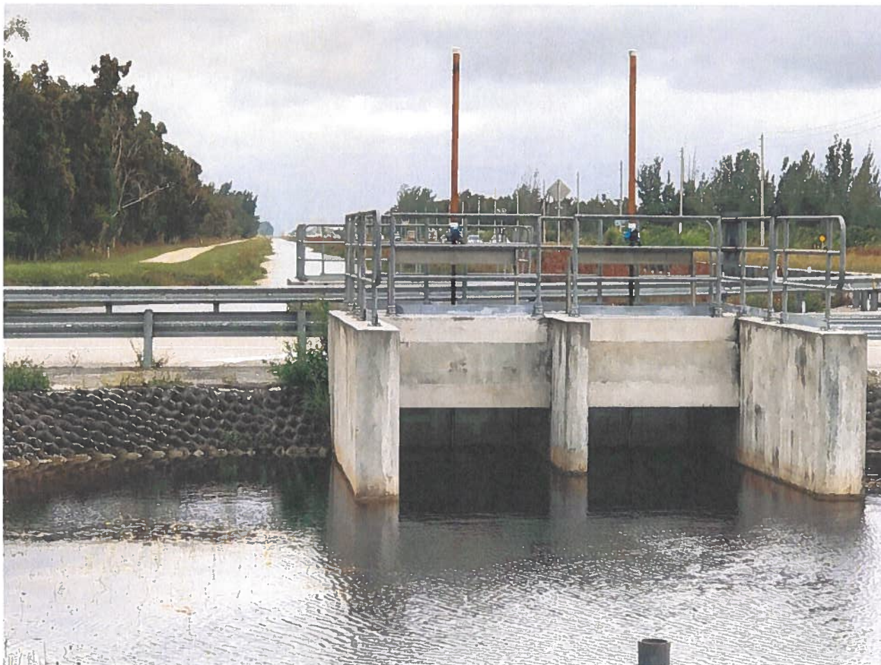
Figure 2: Structure G-119 Upstream View (photo by S. Hajimirzaie 11/09/2019)
