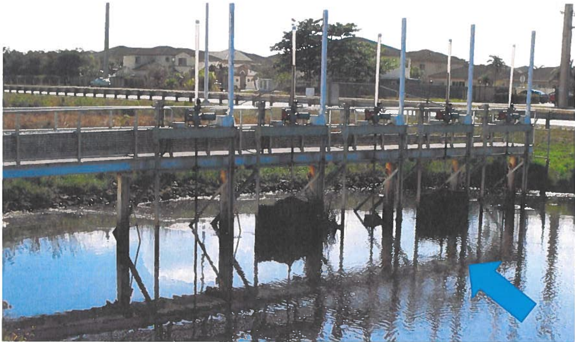
Figure 3: Structure S-380 Upstream (top) and downstream trash rake (bottom) View
