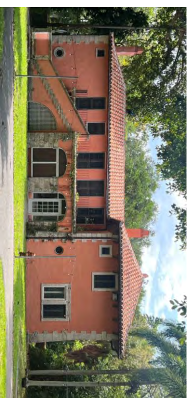
FARM HOUSE PRIOR TO RENOVATION
