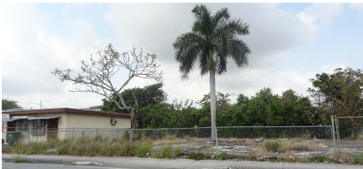
Figure 10: Building and Site Deterioration
