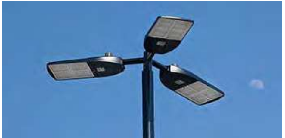
LED Lighting with solar sensors and lens cut-off
