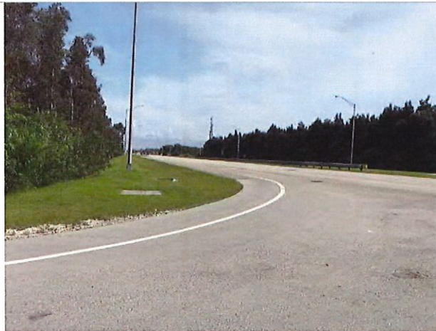
Looking Northward on Krome Avenue
