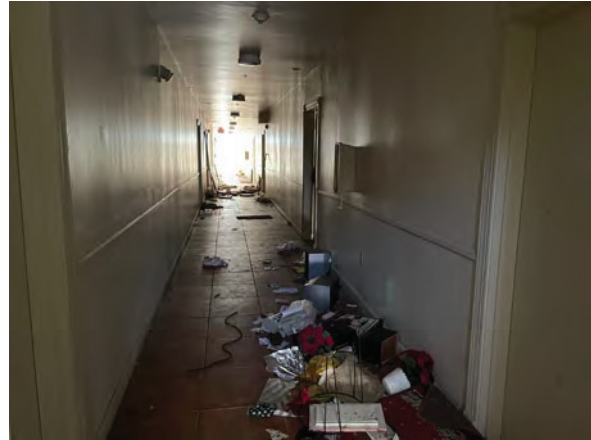
Photo 8 – 3 rd Floor Hallway
