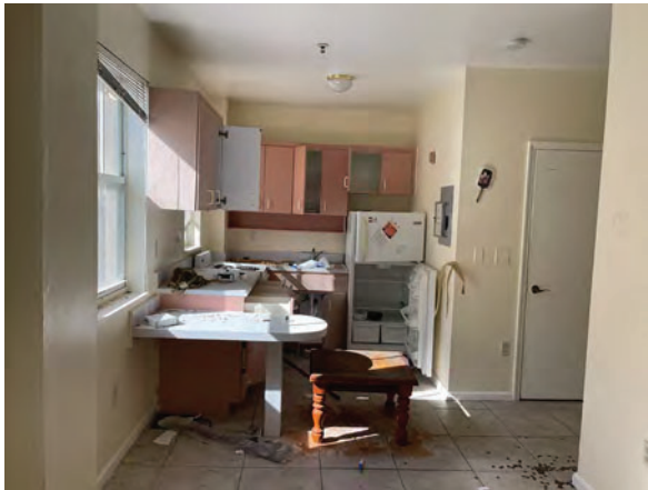
Photo 9 – Typical Kitchen Area
