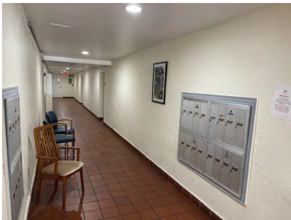
Photo 5 – 1 st Floor Common Hallway
