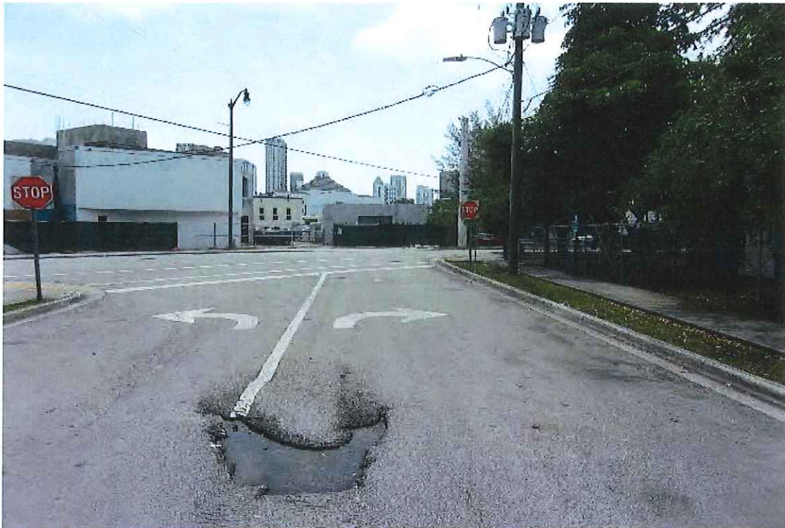
LOOKING EASTERLY ON N. W. 3 RD STREET – SUBJECT TO LEFT
