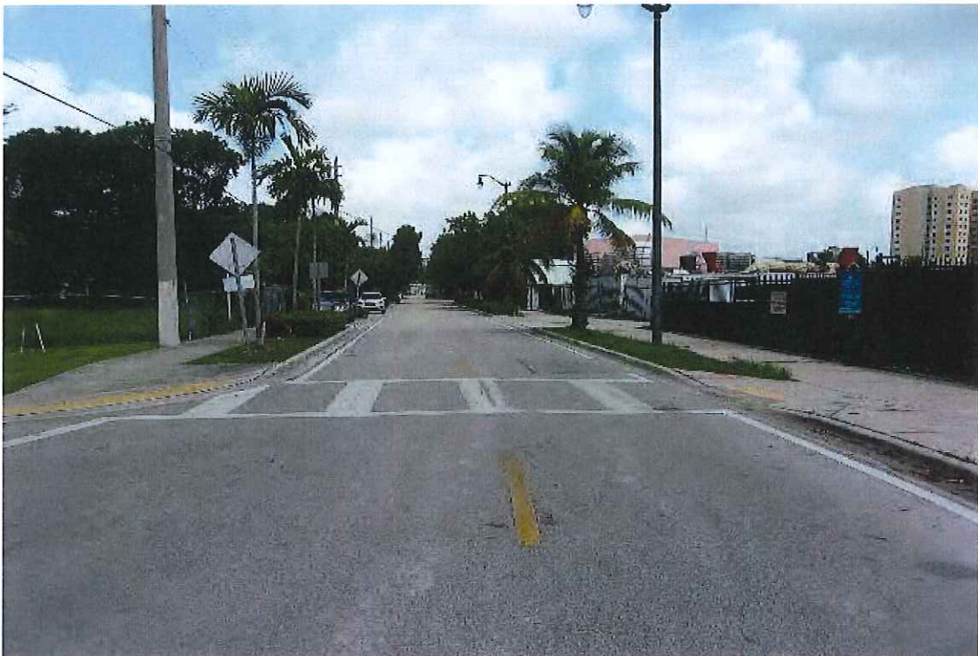
LOOKING WESTERLY N. W. SOUTH RIVER DRIVE ON – SUBJECT TO LEFT
