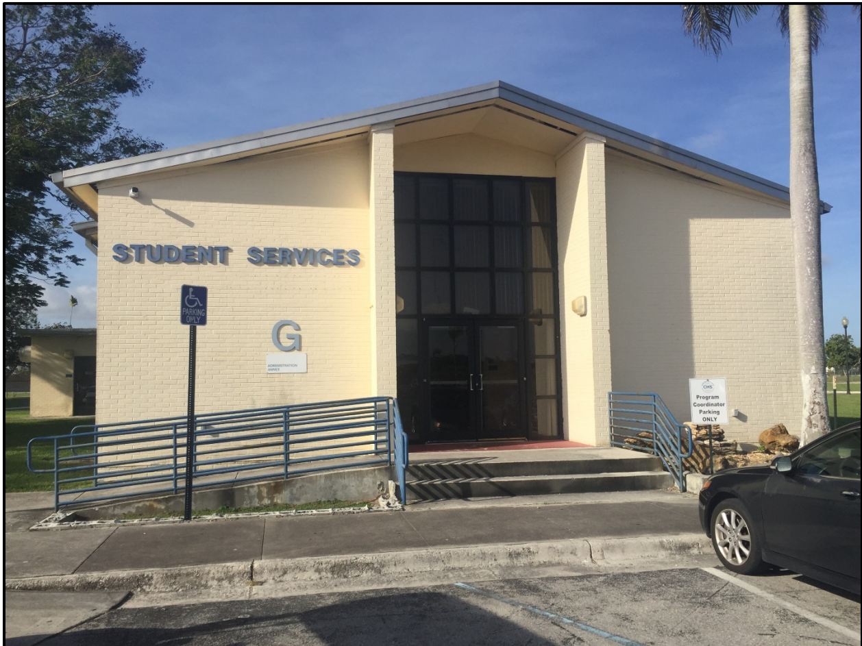
Figure 5. Student Services Building (Building G – Former Chapel), northeast (primary) façade, facing southwest
