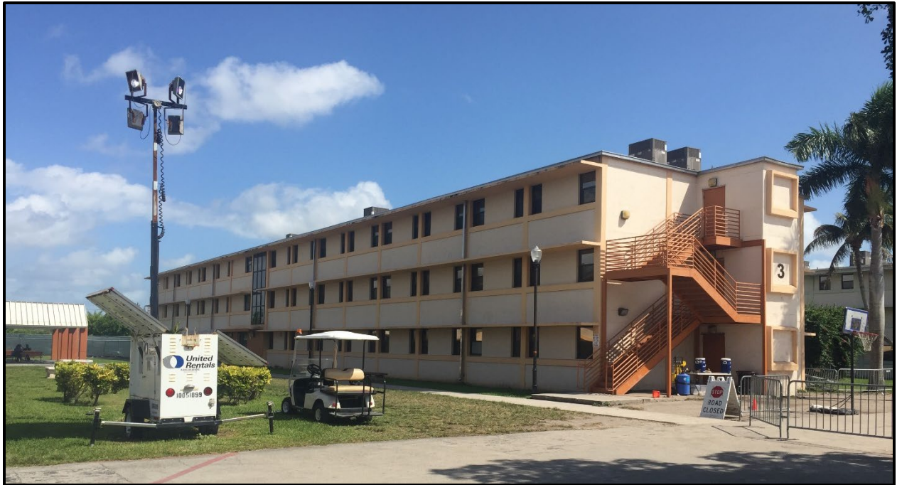
Figure 8. Residence Hall, Building N (Former Barracks), north (primary) and west façades
