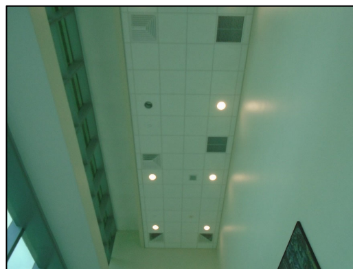
Courthouse Interior Lighting 1
