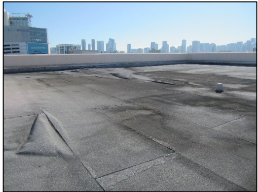
Graham Building Upper Roof 1
