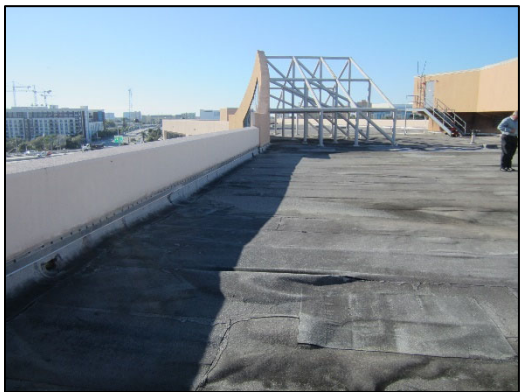
Graham Building Upper Roof 2
