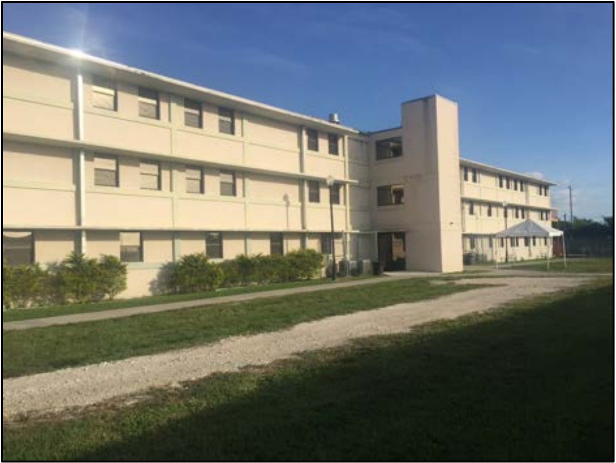
Figure 9. Educational Training Wellness Center, Building O (Former Barracks), south (primary) façade, showing addition of an elevator shaft
