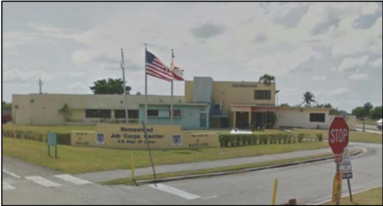
Figure 7. Former Recreation Building (Building J). northwest (primary) façade facing southeast (Google Map data 2019 [May 2011])
