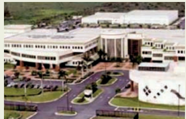
MDPD Fred Taylor Headquarters Building
