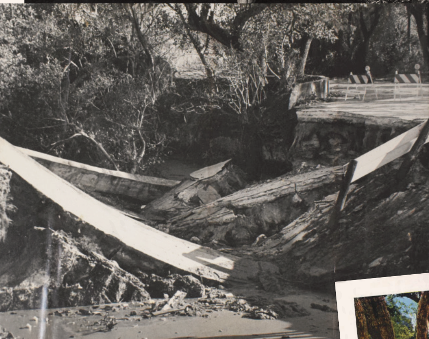
▲ Arch Creek natural bridge collapsed in February 1973.
