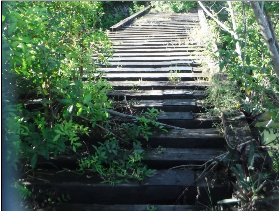
Figure 23: Decking with Wood Rail Ties and Steel Tie Plates, Facing North
