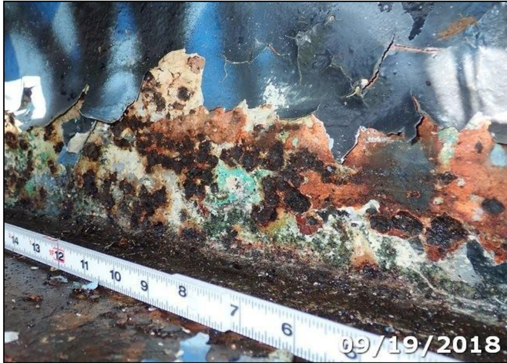
Photo 07: Both beams exhibit severe corrosion throughout with pitting.
