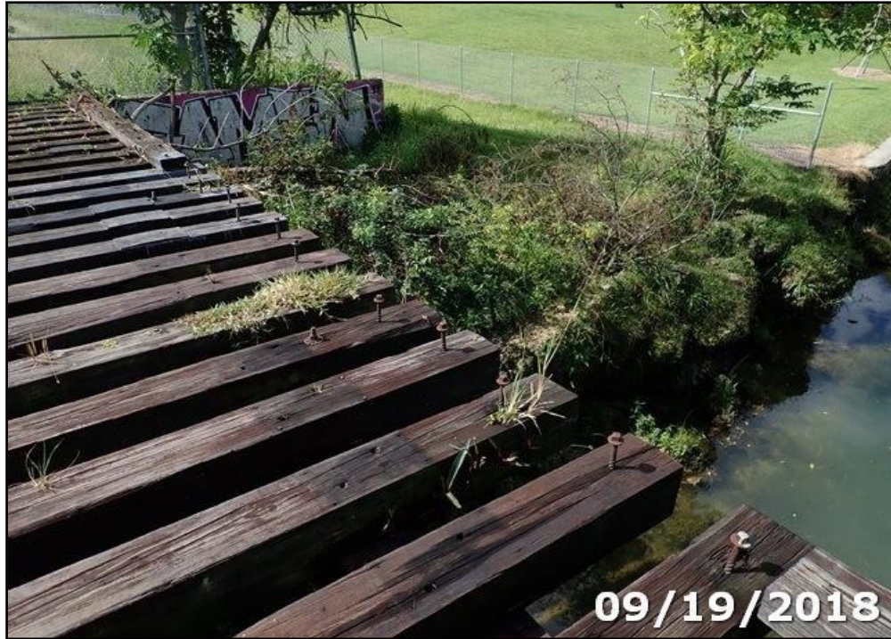
Photo 03: Missing section 16ft. L on the left timber guard at Span 2.
