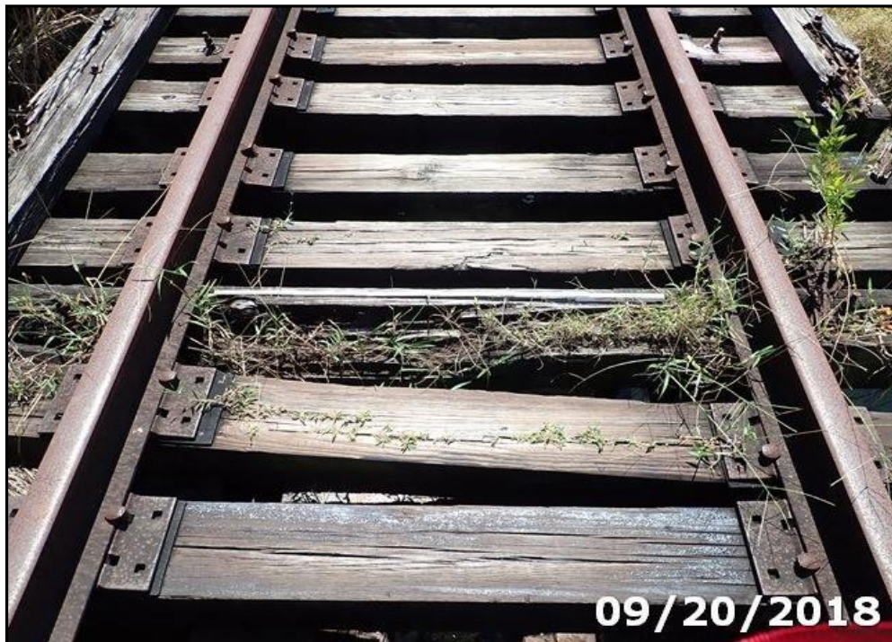
Photo 02: Typical decay with vegetation growth on railroad ties.
