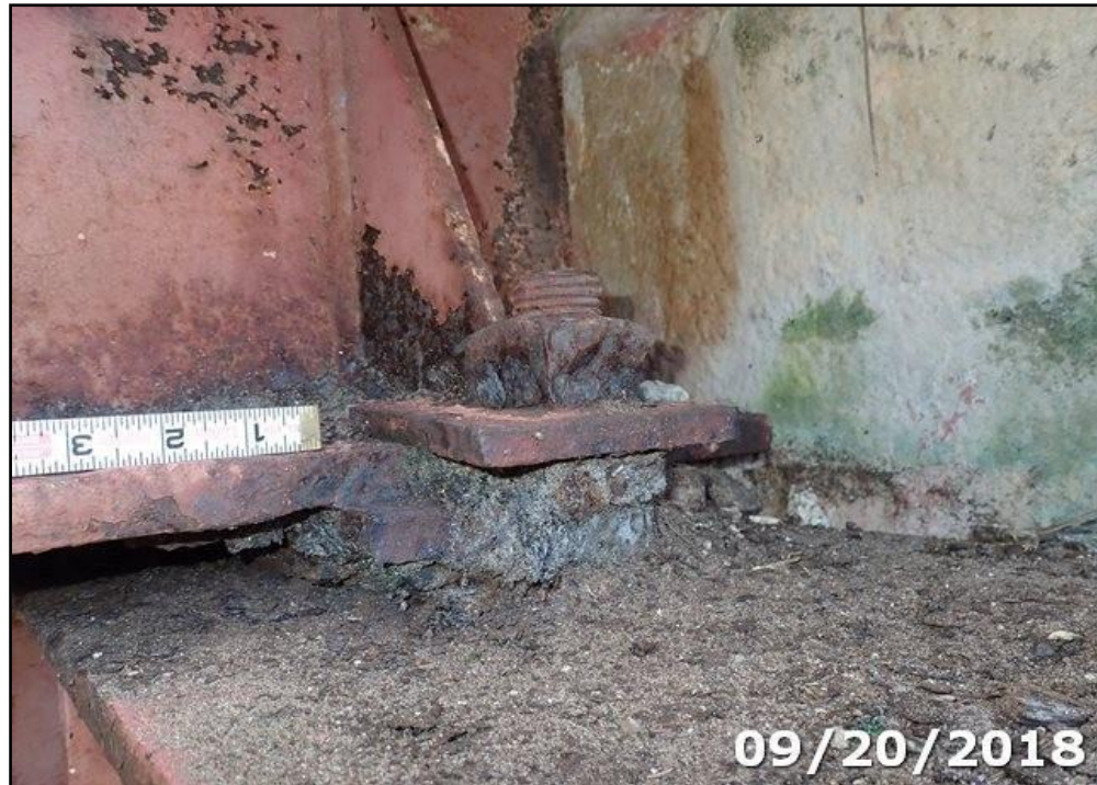
Photo 07: Typical corrosion with section loss up to 50% on the bearing plates and anchorage hardware.
