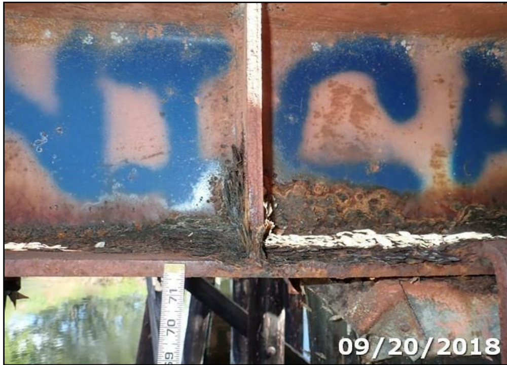
Photo 09: Severe corrosion with up to 40% section remaining on the steel pier caps. There is graffiti on the faces of the pier caps. Shown Pier cap 3, south face.
