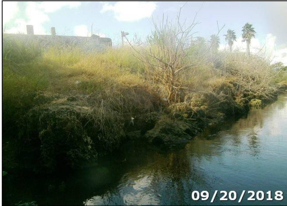
Photo 19: The channel embankments exhibit erosion at both sides of the bridge.
