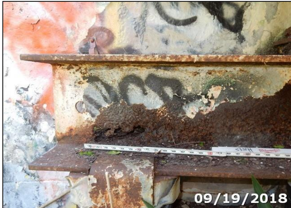
Photo 13: Severe corrosion with section loss up to 100% at east end of Abutment 1 cap. (Front view)
