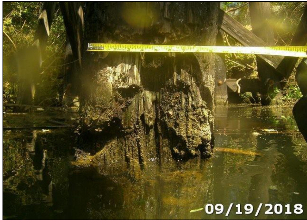
Photo 19: Typical decay on the piles of Bents 3 thru 6 at the tide zone.
