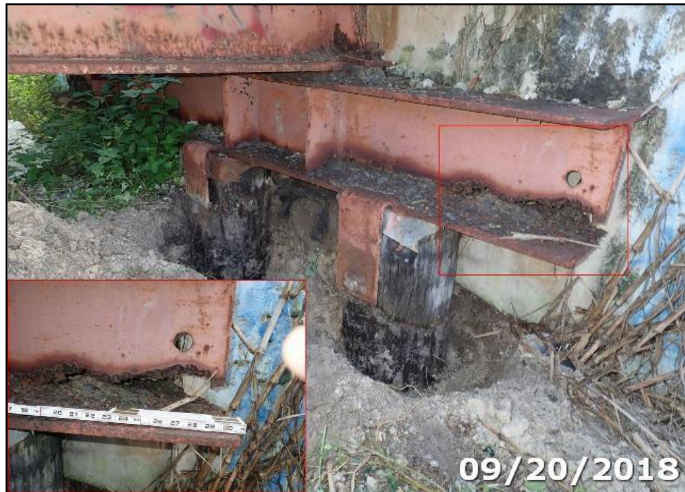
Photo 10: Severe corrosion on the webs and bottom flanges of the abutment caps with up to 100% section loss at the ends.
