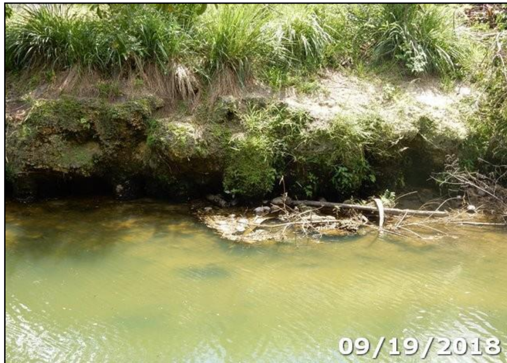
Photo 24: Typical erosion at the channel slopes.
