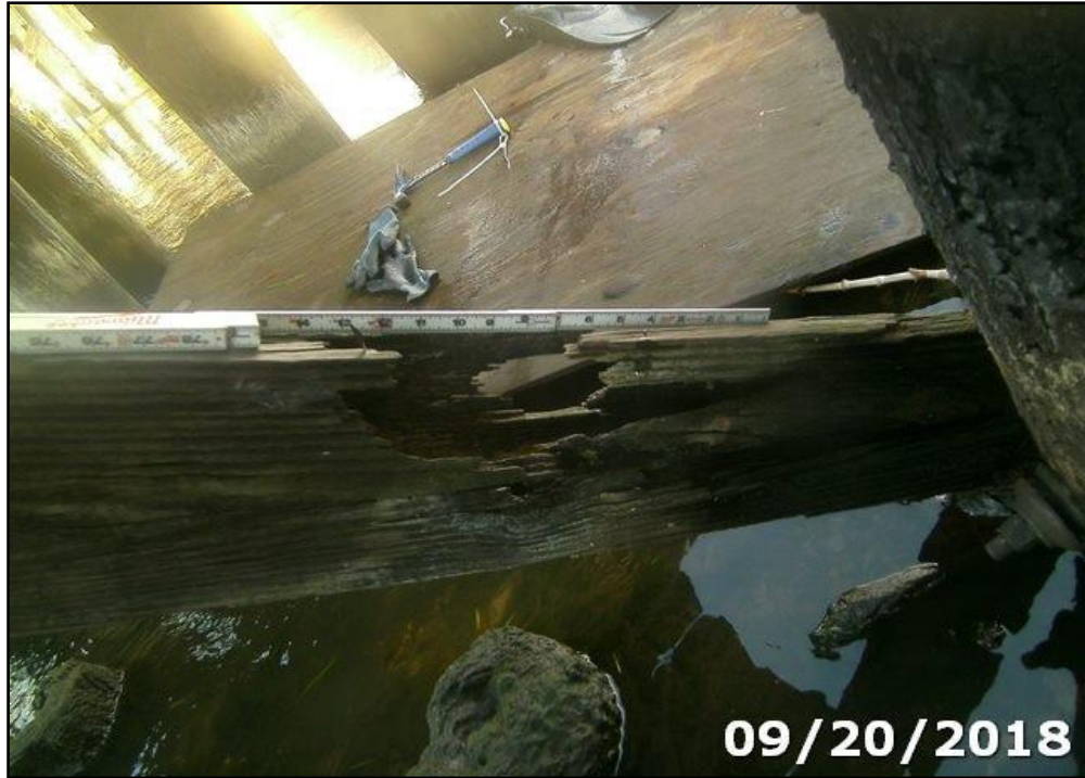
Photo 17: The cross bracing members exhibit areas of severe decay with up to 0% section remaining at the bottom ends.
