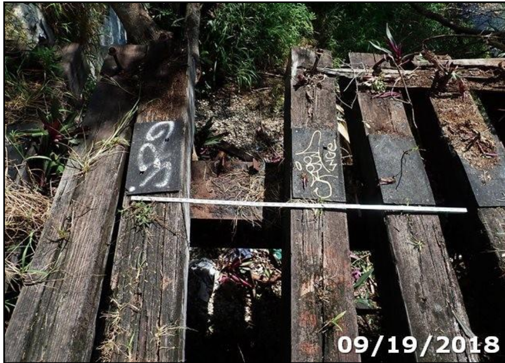
Photo 01: The right (east) timber guard is decayed up to 100%, having the north end missing. The 4th railroad tie from the north is not attached and displaced.
