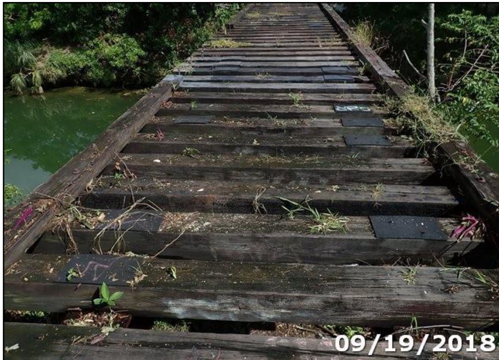
Inventory Photo 02: Timber Deck Overview (Railroad Ties and Timber Guards)
