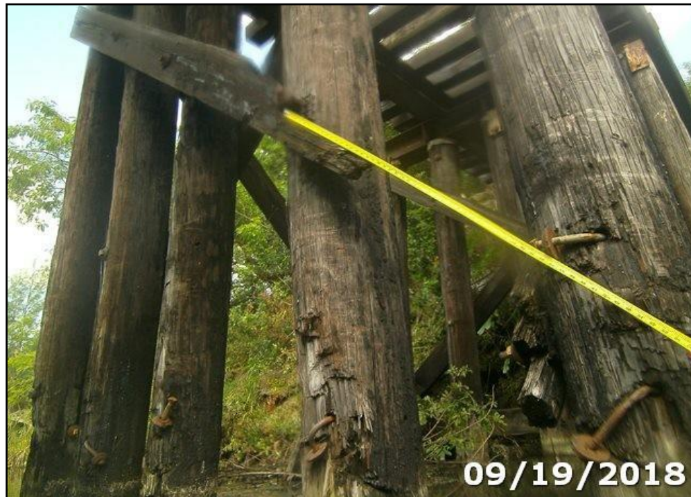
Photo 20: Pier 6 has one broken cross bracing at Pile 6-4, and the horizontal is missing.
