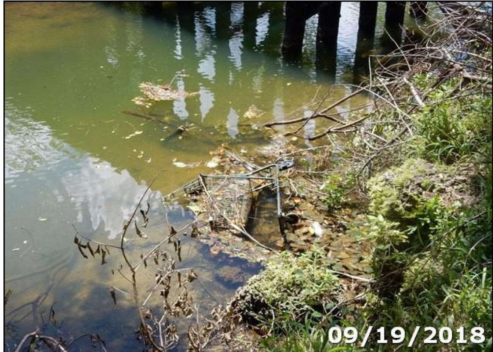
Photo 25: There is drift and debris scattered on the channel.
