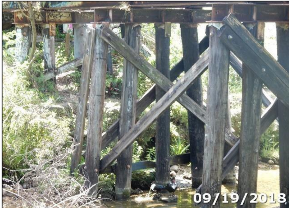
Inventory Photo 07: Typical Timber Piles and Cross Bracing
