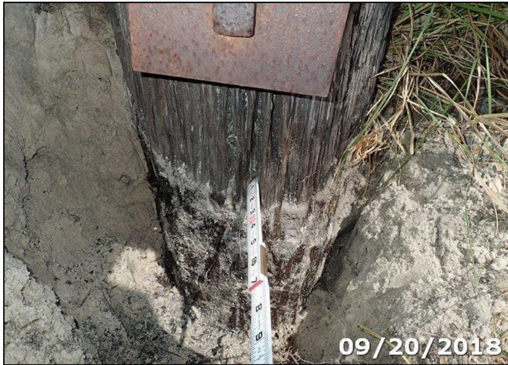
Photo 13: The timber piles typically exhibit checks and splits, and below the groundline have decay with soft areas up to 1-1/2in. D.
