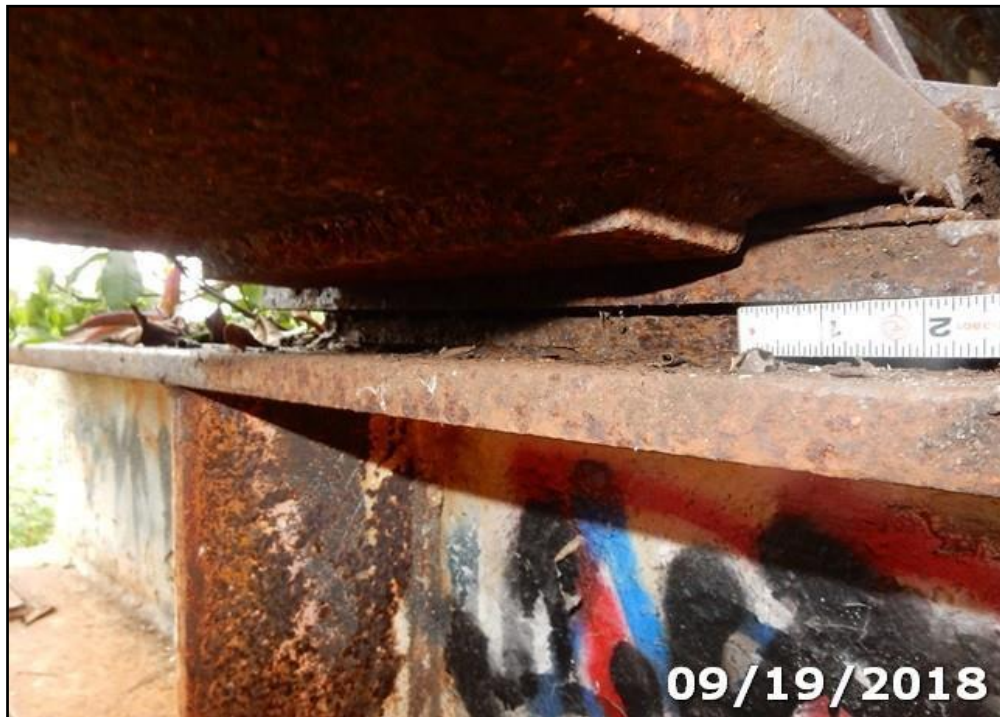
Photo 10: Typical corrosion with pitting at the intermediate bents bearing plates.
