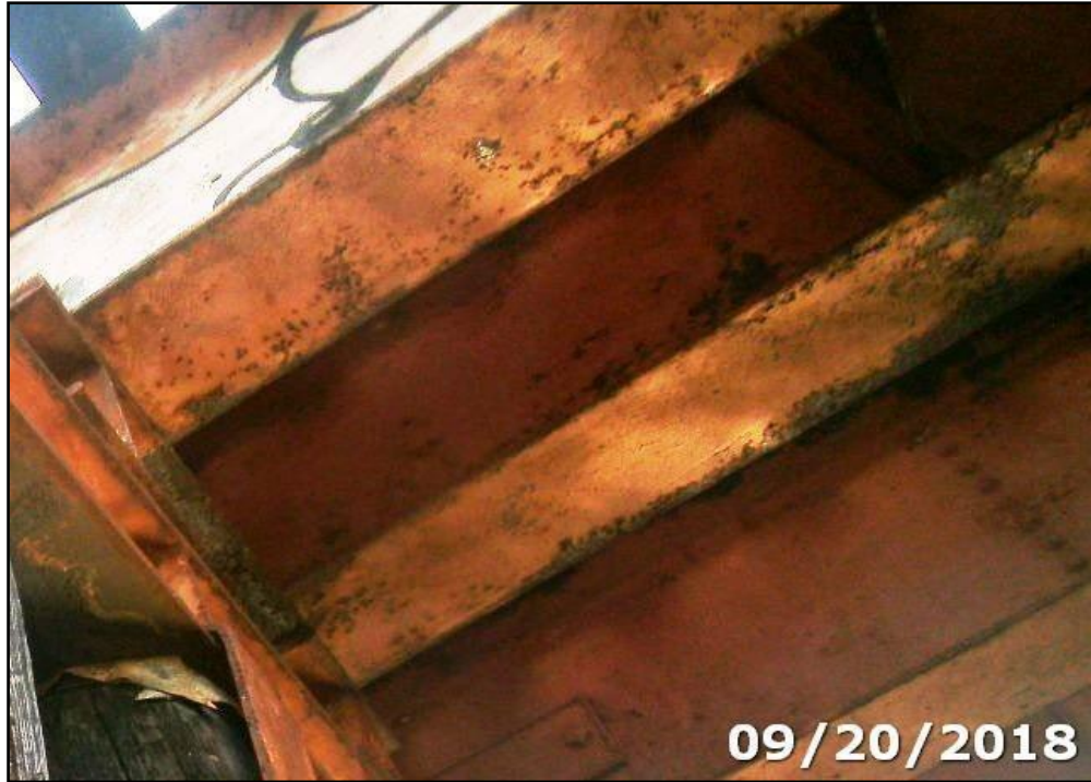
Photo 05: Typical corrosion on the bottom flanges of the steel beams.
