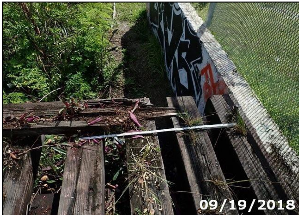
Photo 02: Decayed and missing south end of the right (east) timber guard.
