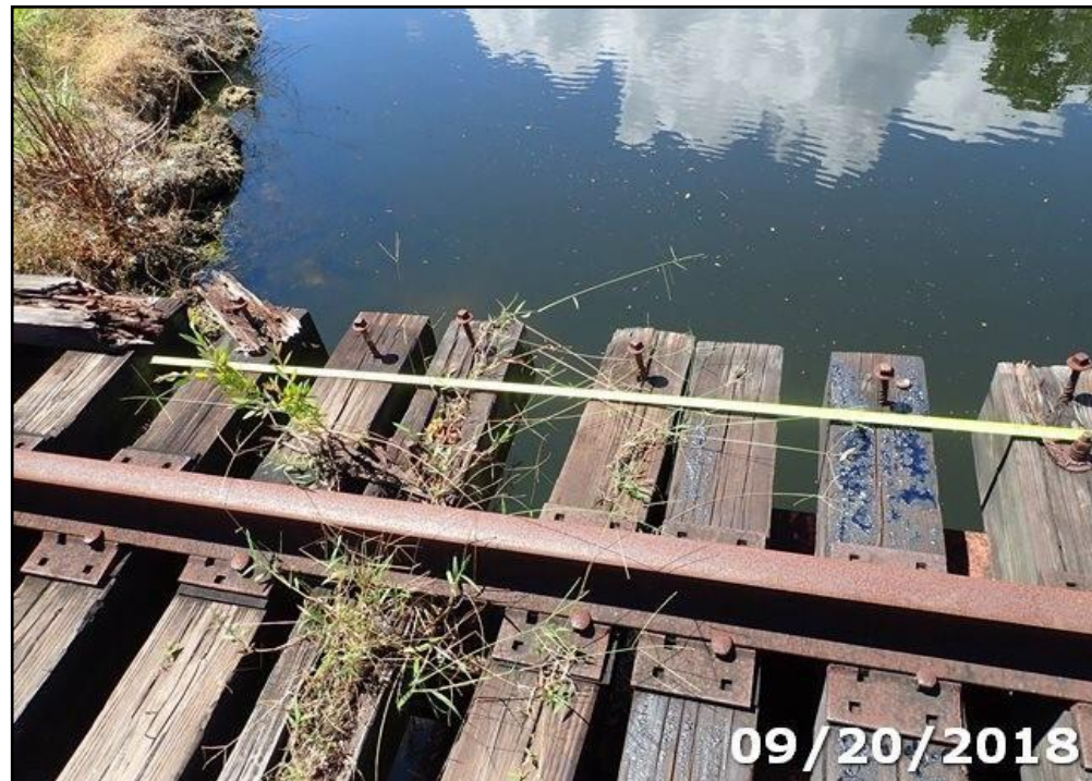
Photo 04: Severe decay and missing sections of the timber guards at both sides of the deck.
