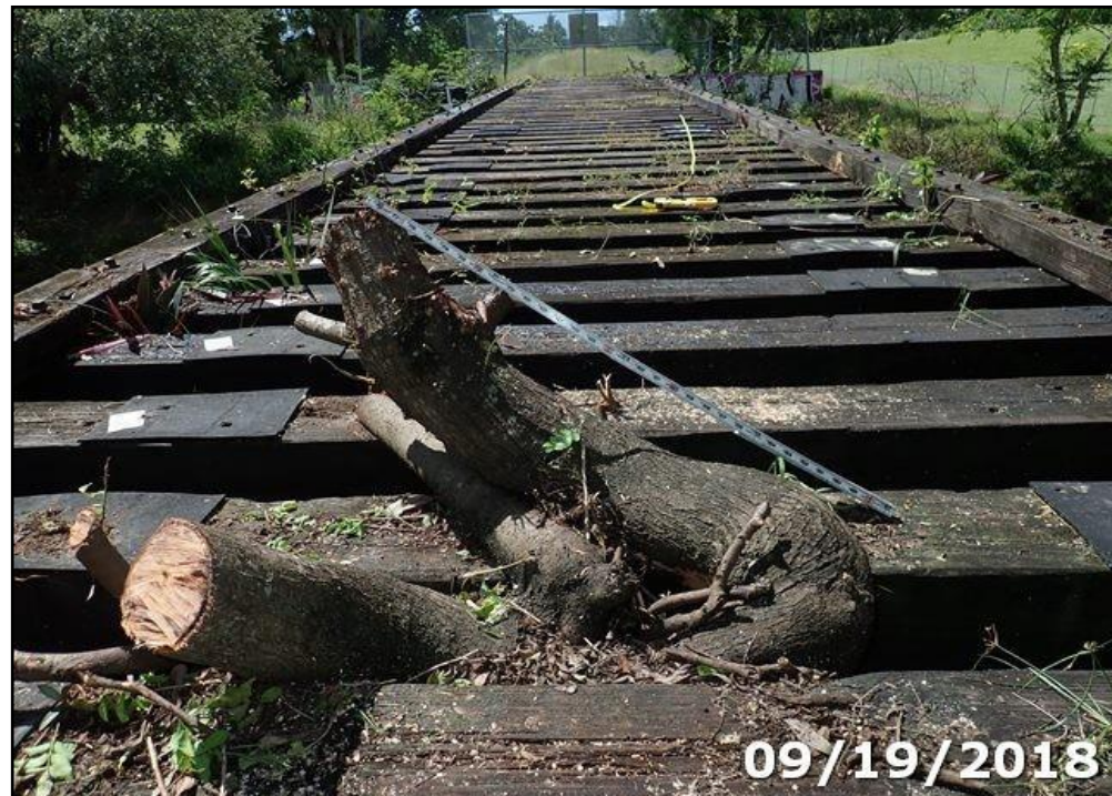
Photo 06: There is a tree growing between the railroad ties at north of Bent 7.
