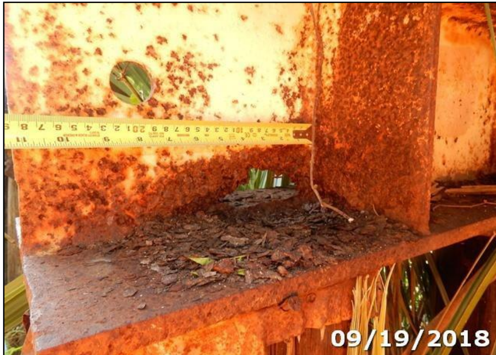
Photo 11: All steel caps exhibit moderate to severe corrosion, having areas of up to 100% section loss at random locations. Shown Pier cap 7, east end.
