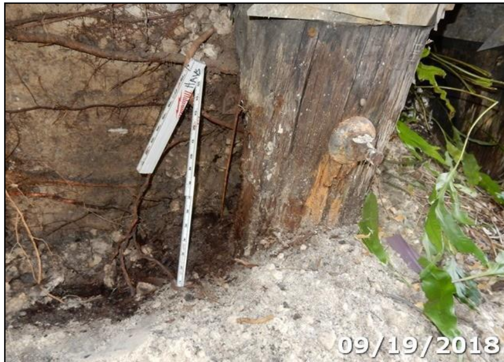
Photo 16: Severe decay with section loss up to 40% below the groundline on Pile 1-2.
