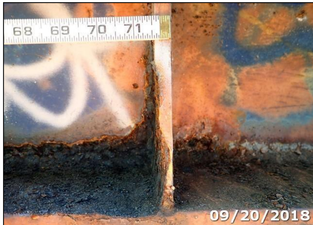
Photo 08: Severe corrosion with up to 40% section remaining on the steel pier caps. There is graffiti on the faces of the pier caps. Shown Pier cap 2, north face.
