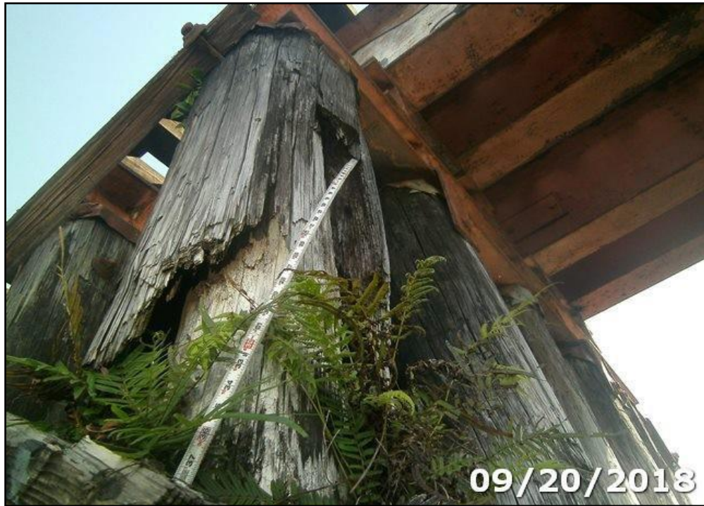
Photo 15: Piles 6-1, 6-3, 6-11, and 6-12 exhibit severe decay and insect activity with up to 20% section remaining. Shown Pile 6-11.
