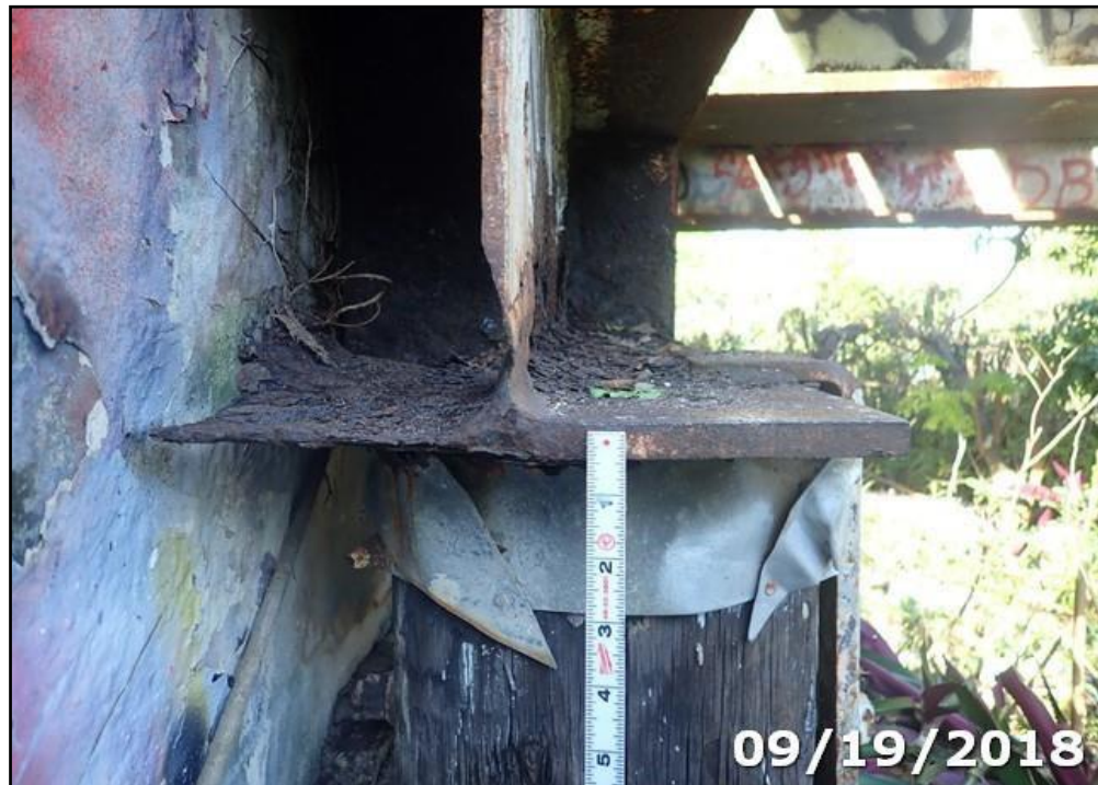
Photo 14: Severe corrosion with section loss up to 100% at east end of Abutment 1 cap. (East view)
