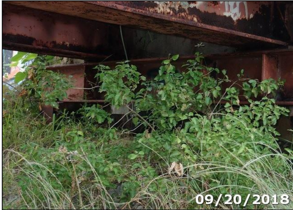
Photo 21: Heavy vegetation growth at both channel slopes below the structure.
