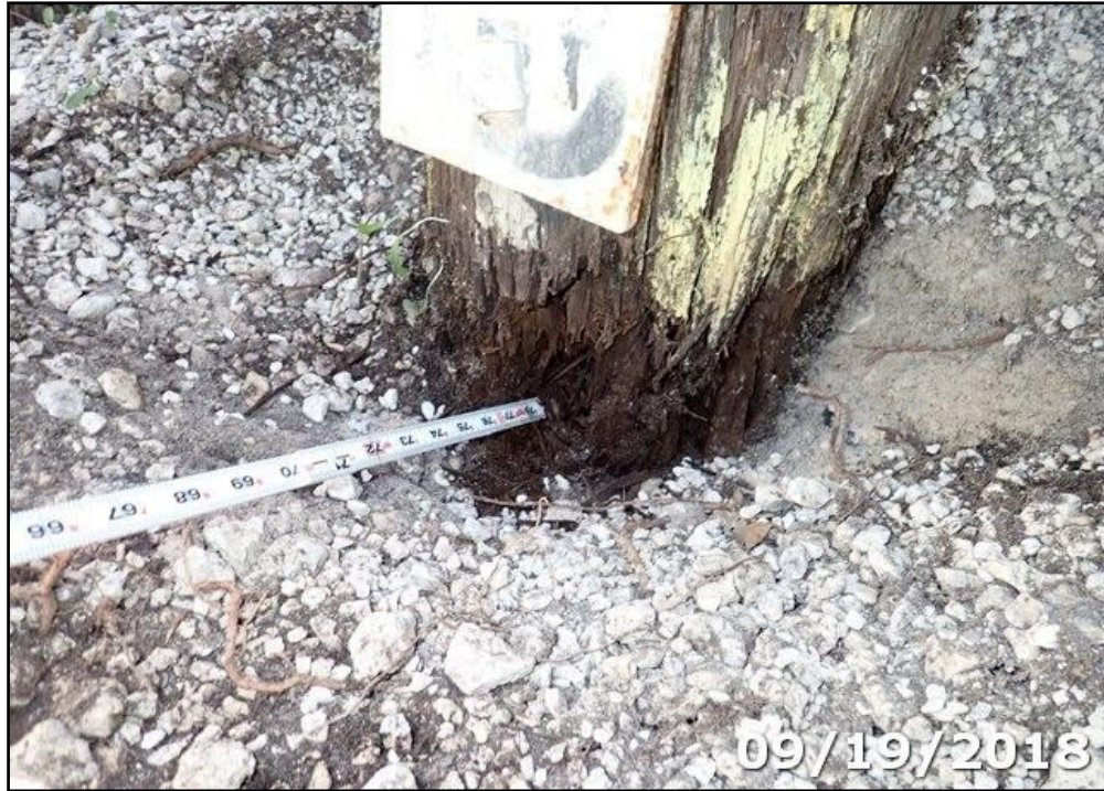
Photo 15: Pile 8-3 exhibits severe decay with section loss up to 70% below the groundline.
