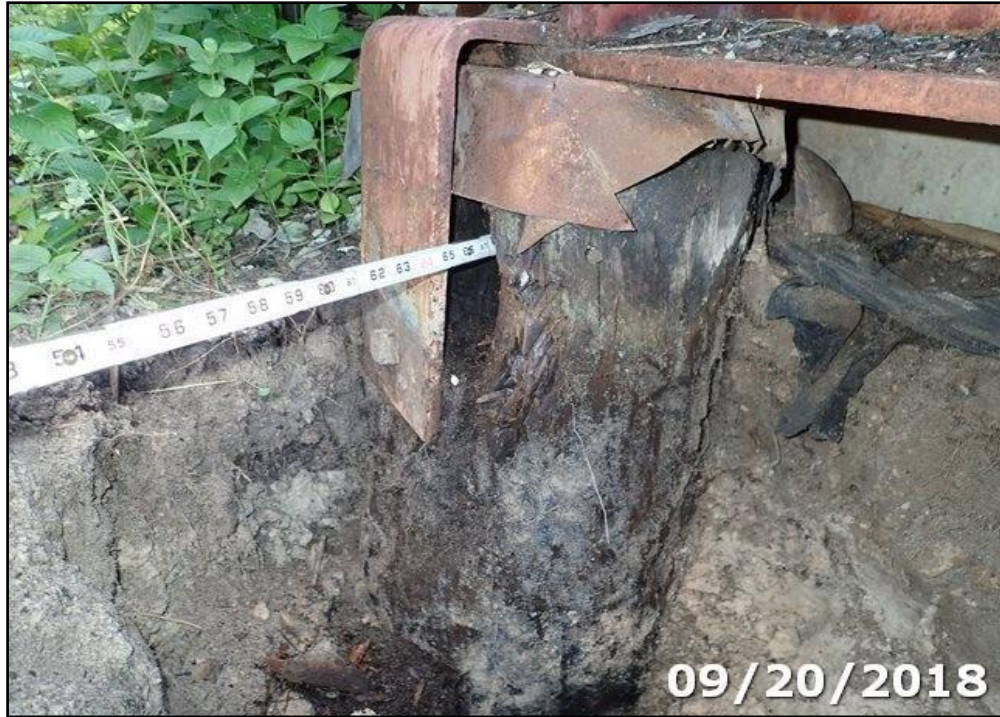
Photo 11: Severe decay with section loss at the top of the timber piles. Shown Pile 1-2.
