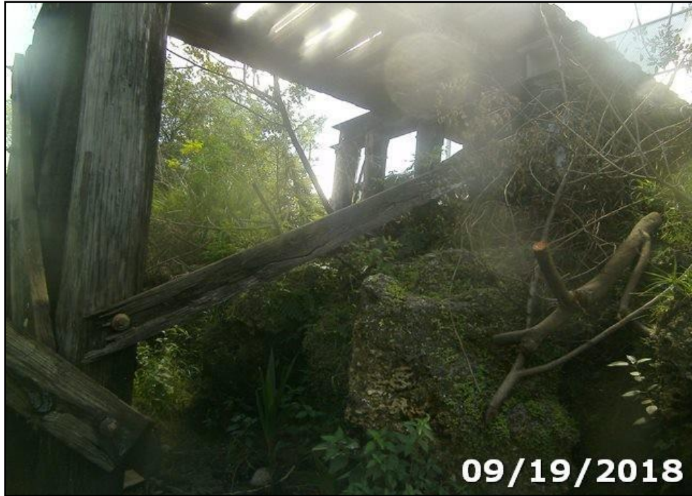
Photo 21: Typical decay with section loss at the bottom ends of the cross bracing members.
