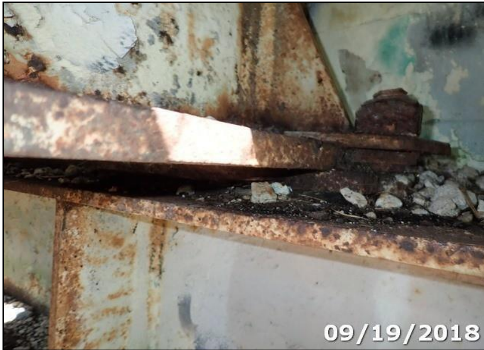
Inventory Photo 05: Typical Elastomeric Bearing
