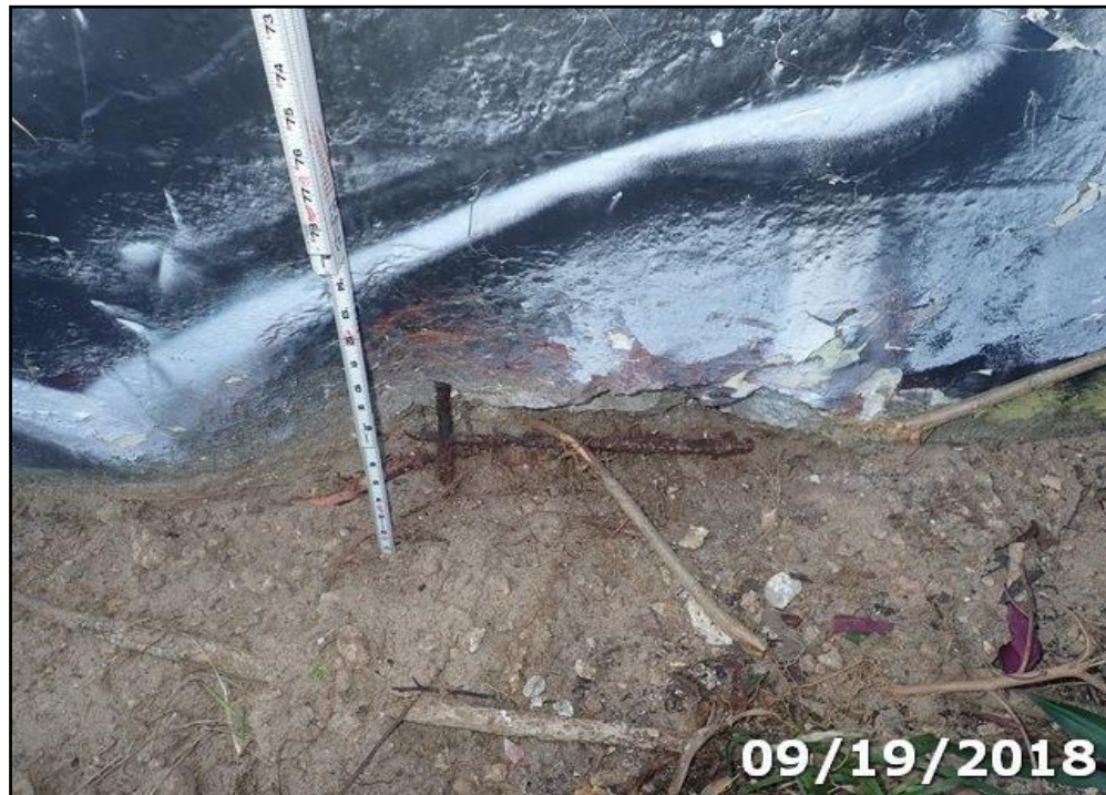
Photo 22: Spall 30in. L x 15in. H x 3in. D with two exposed rebar at Abutment 1 concrete wall, 2ft. west of Pile 1-5.
