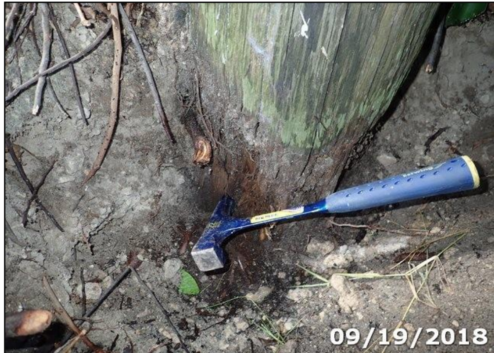
Photo 17: Severe decay with section loss up to 50% below the groundline on Pile 2-3.
