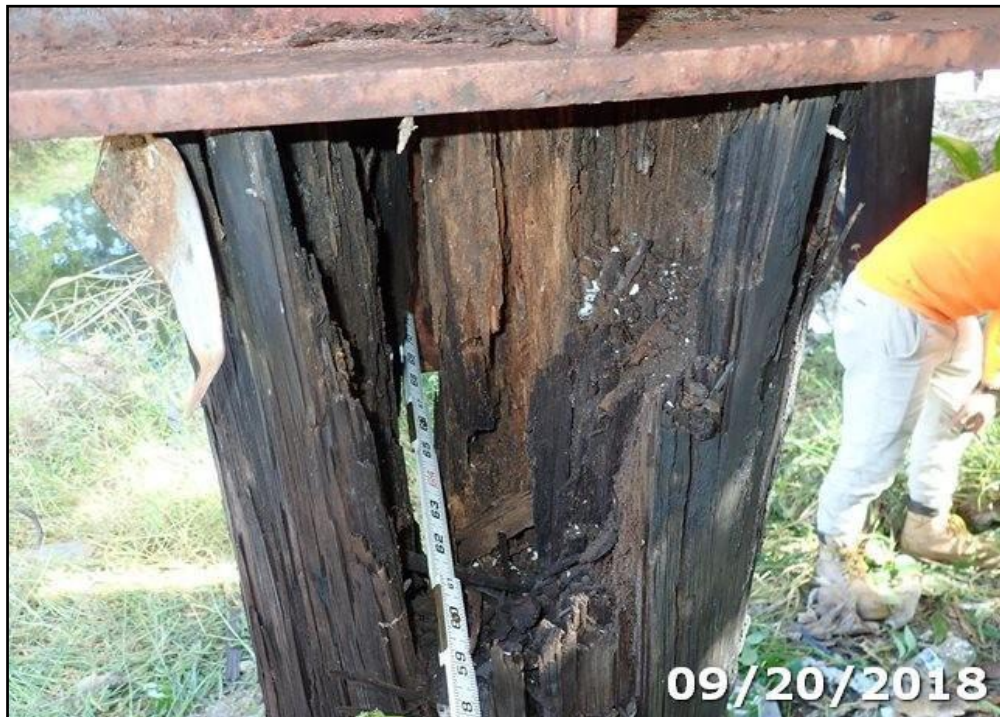
Photo 12: Severe decay with section loss at the top of the timber piles. Shown Pile 2-1.
