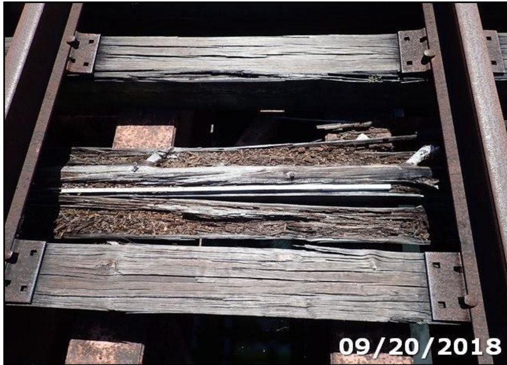
Photo 01: Typical splits and checks on railroad ties. Severe decay at Ties 10, 11, 22 ,28, 29, 30, 40, 41, 44, 49, 52, 53, 54, 69, 71, 76, 79, and 80.
