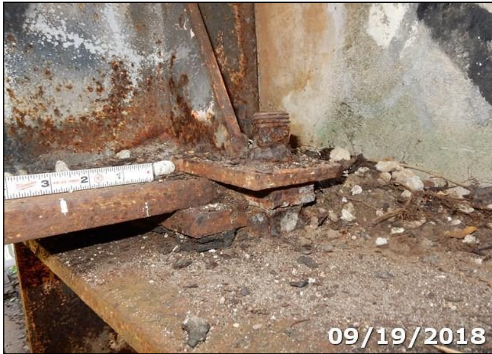
Photo 09: The bearing plates and anchorage hardware are heavily corroded with up to 100% section loss. Neoprene pads at abutment bearings.
