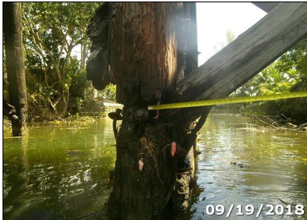
Photo 18: Pile 4-1 and the cross bracing have severe decay, having up to 100% section loss at the cross bracing connection.
