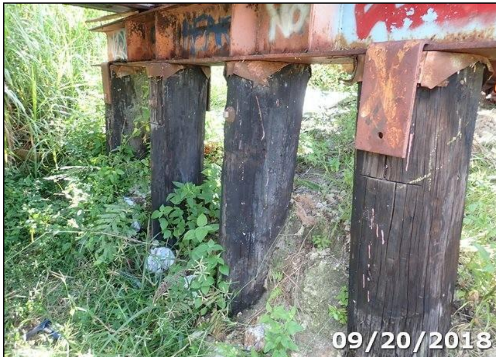
Photo 16: The timber piles at Bents 2 and 3 exhibit minor fire damage.
