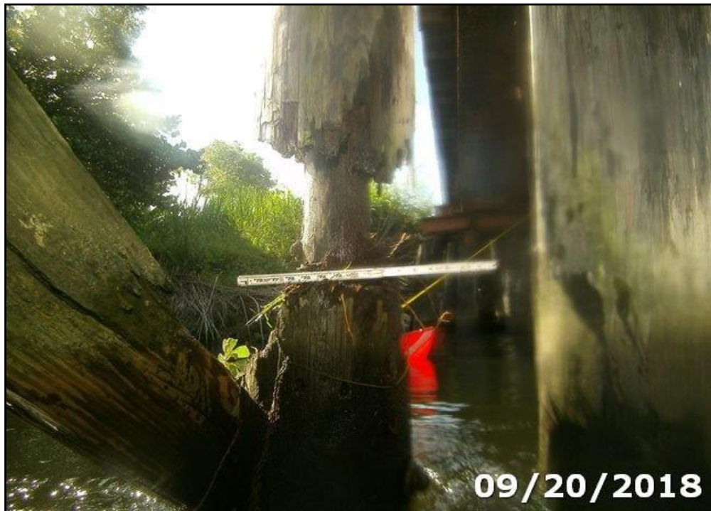
Photo 14: Piles 6-1, 6-3, 6-11, and 6-12 exhibit severe decay and insect activity with up to 20% section remaining. Shown Pile 6-1.
