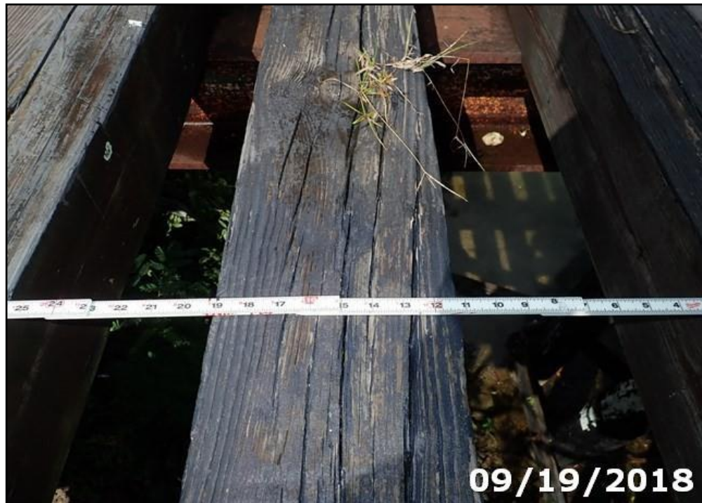
Photo 04: Typical splits and checks on the railroad ties.
