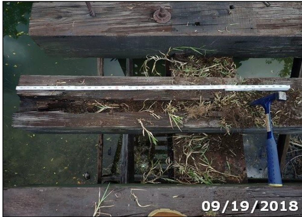
Photo 05: Typical severe decay and vegetation growth on some railroad ties.
