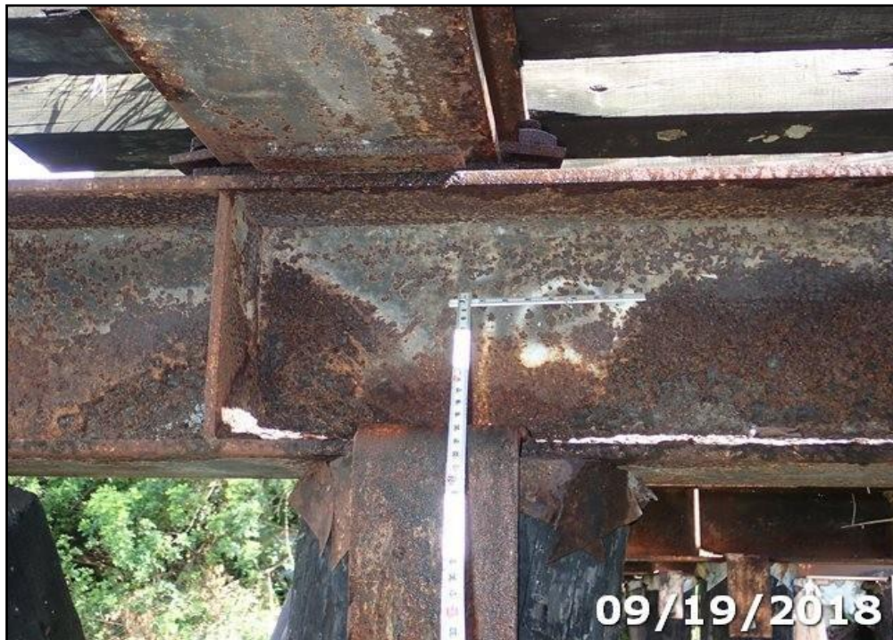
Photo 12: Typical corrosion with pitting on the steel pier caps.
