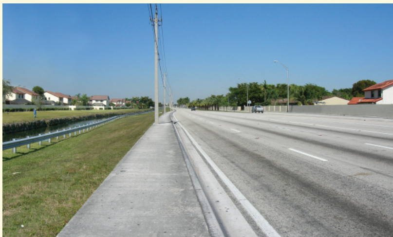
SW 137th Avenue - Existing
