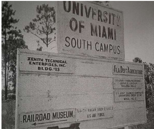
Signage for Zenith Technical Enterprises, 1964. (Castro Obsession, photo section)
