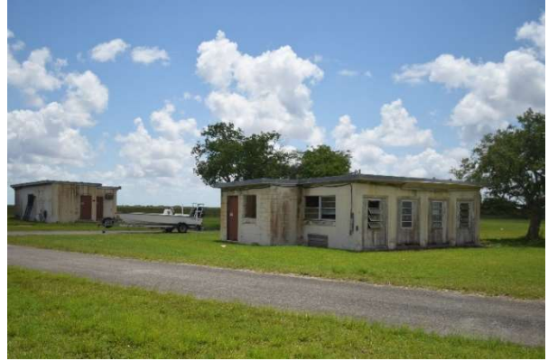
Interconnecting Connecting Building and Generator Building, 2019.
