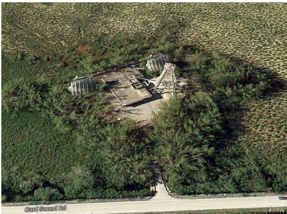
Aerial view of Microwave Tower site, 2019. (Imagery ©2019 Google, Map data ©2019)
