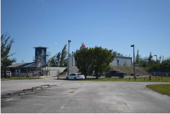
View of HM-39, looking south, 2019
