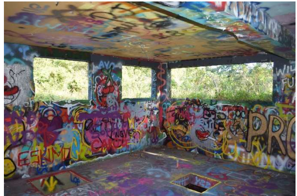
Interior of Observation Station, 2019.
