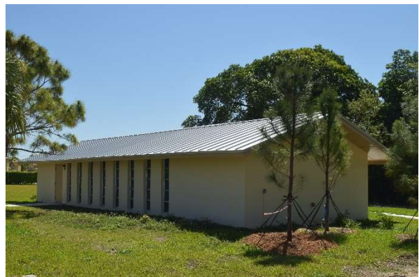
Building at Camp Matecumbe, 2019.
