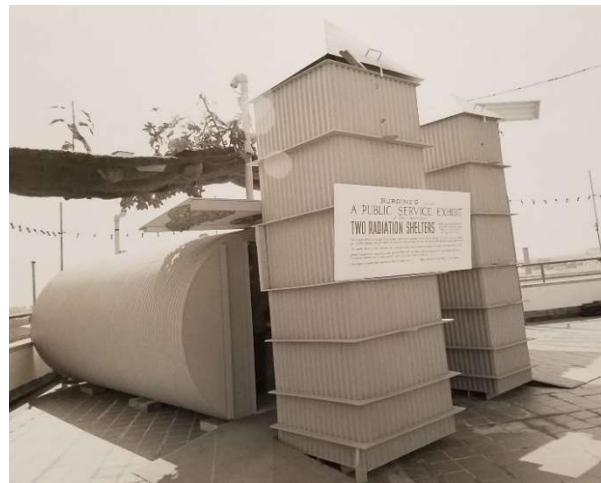
Radiation shelters displayed on top of Burdine's Department Store, 1961. (HistoryMiami Archives)
