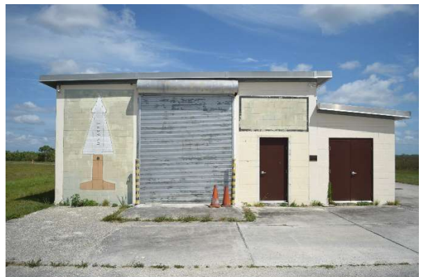
Missile Assembly and Warheading Building, 2019.
