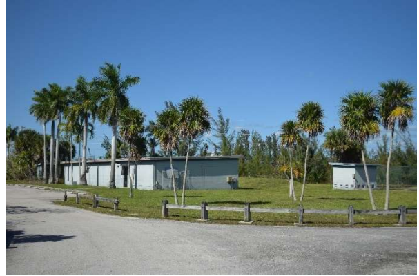
View of HM-39, looking northeast, 2019.
