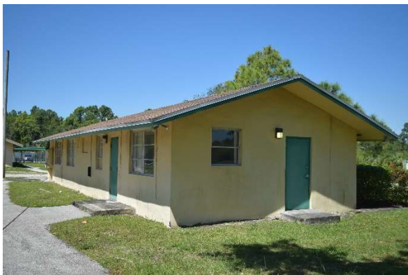
Building at Camp Matecumbe, 2019.
