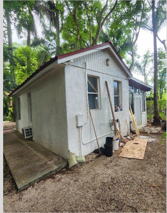
Rear of Caretaker's cottage, 2023
