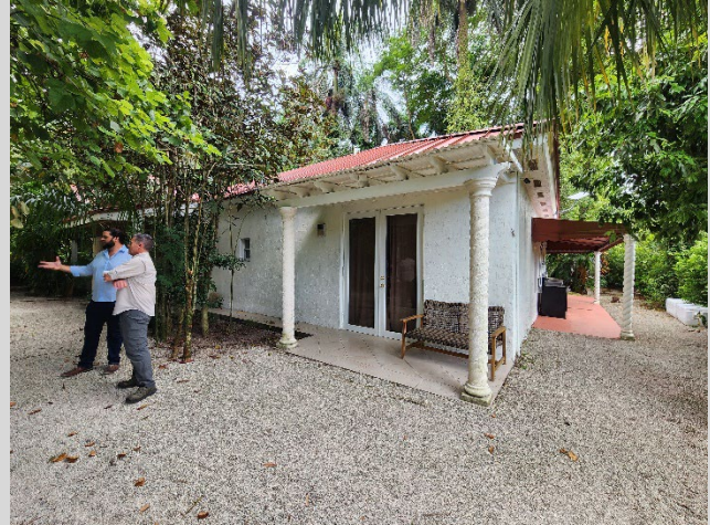
North Façade with porch addition, 2023
