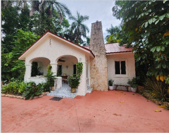
East Façade - Courtyard , 2023
