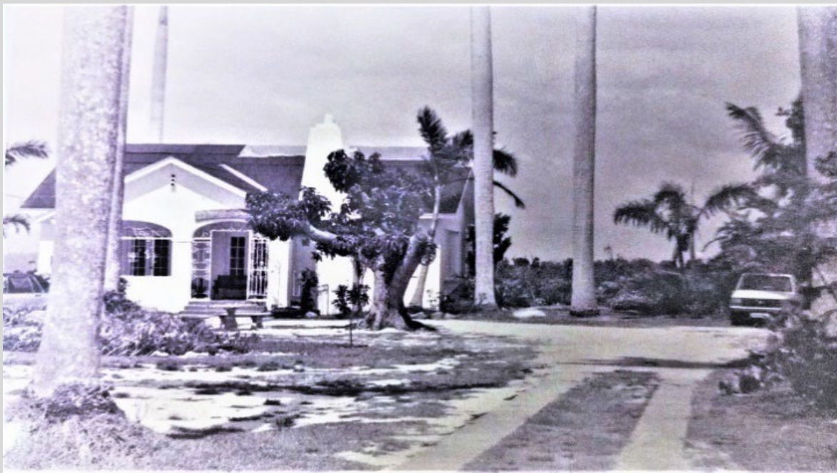
Front (east) Elevation ca. 1993
