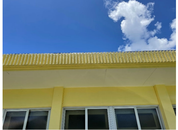
Close-up view of Boystown Dormitory dentil molding.
