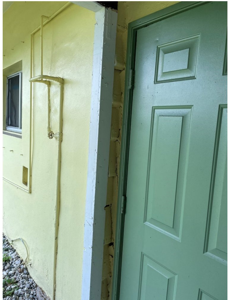
Corner of the building, under the canopy, with wood siding exposed.
