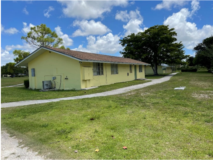
View of Dormitory Number 6 from south.
