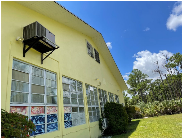
Close-up view of Gym/Multipurpose Building from north.
