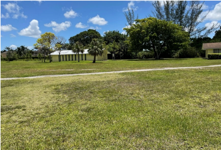
View of Chapel and part of Dormitory Number 6 from north.
