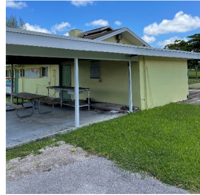
Canopy/outdoor dining area, kitchen extension, and mid-century dovecote on roof.
