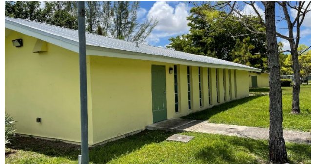
View of Chapel from south.
