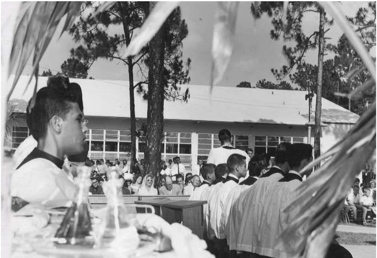
Gym/multipurpose building c. 1962 photographed in 1962 showing window pattern that continues today and showing a ceremony including Pedro Pan Children. 30
