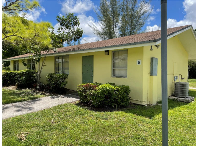
View of Dormitory Number 6 from north.
