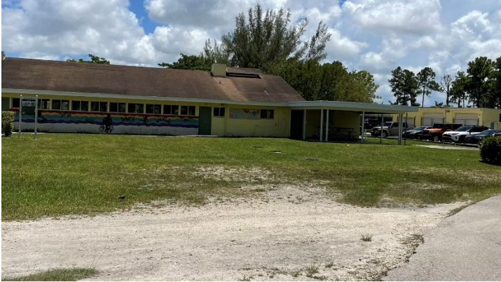
View of Dining Hall Building from the north.
