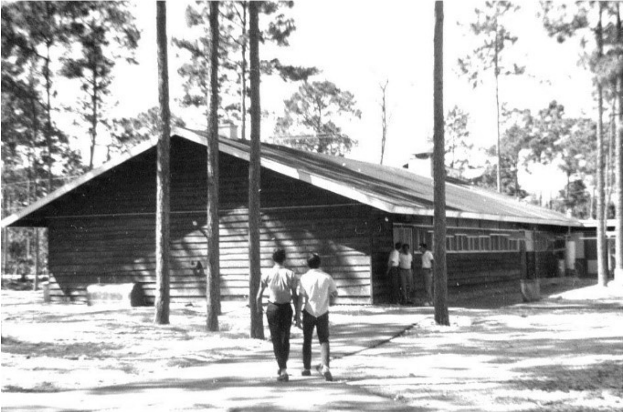
Dining Hall c. 1956, photographed in 1962 showing wood siding, trees in vicinity, and children from Operation Pedro Pan. 29
