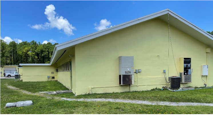
View from west of south façade.
