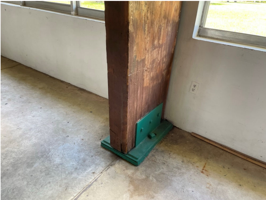
Close-up view of arched truss base plates.
