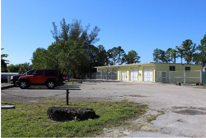
View of Maintenance Building from west (photo: https://rs.locationshub.com/Home/LocationDetail?rsLocationId=029-10000432 ).
