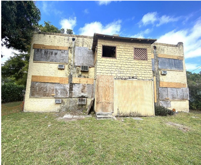
View of South Façade with projecting two-story lanai (2025)
