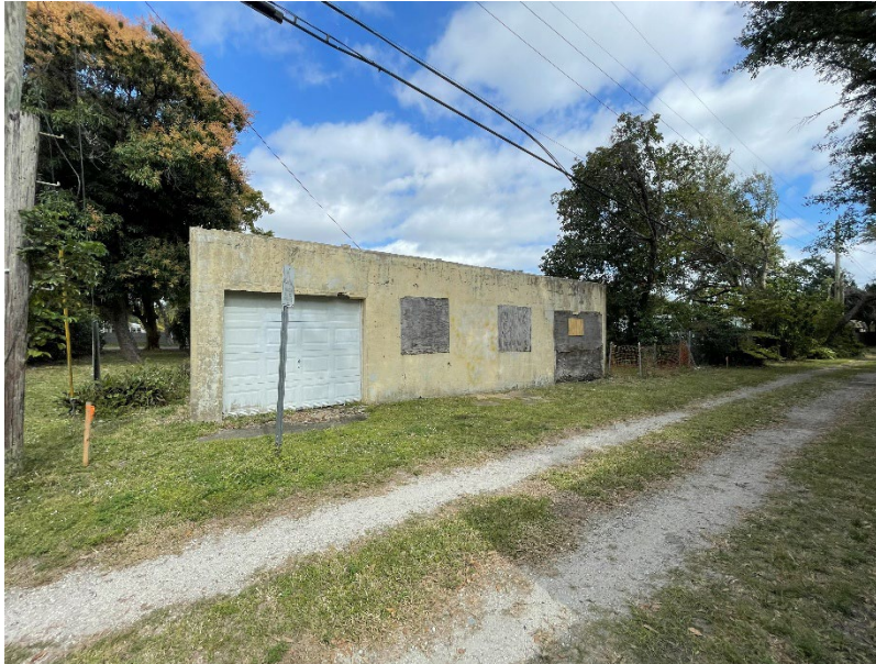
View of Garage and rear access road to property (2025)
