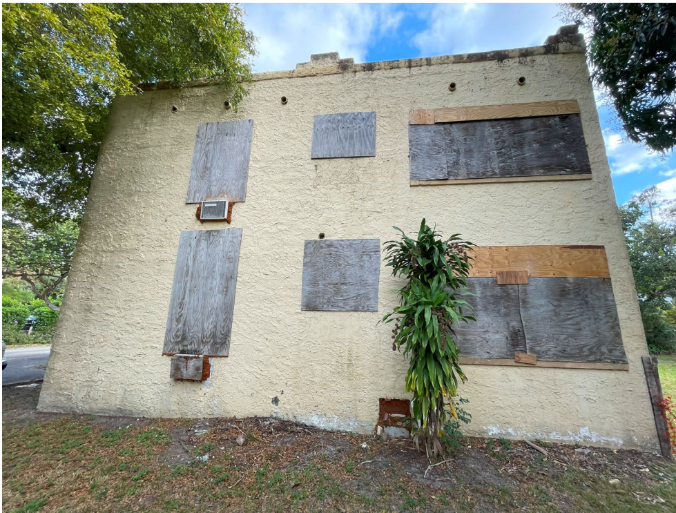
View of West Façade (2025).
