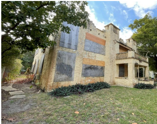
View of the North façade with partial view of East Façade with a pavestone walkway visible. (2025)
