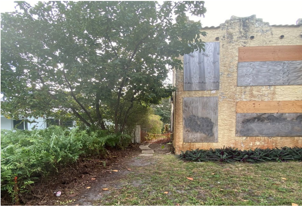
Easternmost end of the North façade with pavestone walkway at east façade visible (2025).
