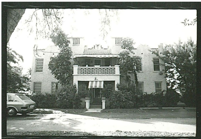
Photograph of primary structure, looking towards the north façade from NE 121 st
