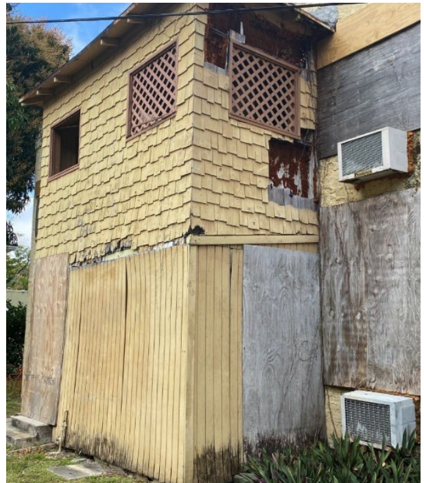
South façade Lanai featuring cedar shake siding and lattice wood screened windows. (2025)
