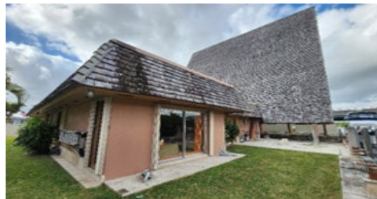
View of North Façade/Rear Entrance, 2023
