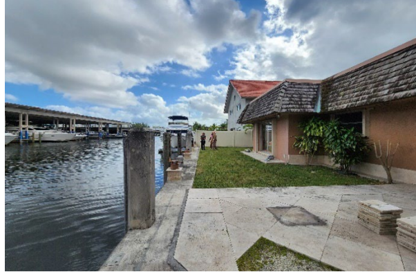
View from North elevation of canal access
