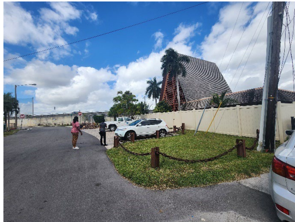
View looking west with subject property at (left) and NW 37 th Street Bridge ahead with ornamental wood and chain cage visible.
