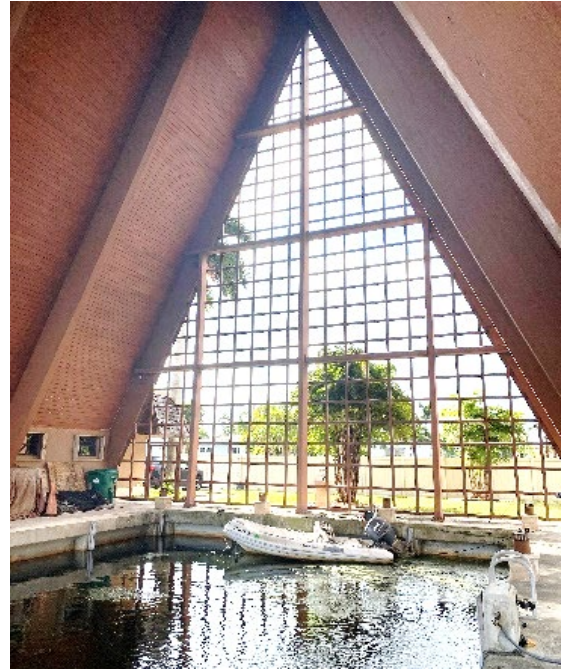
Looking south toward the Boathouse façade from within its interior, 2023
