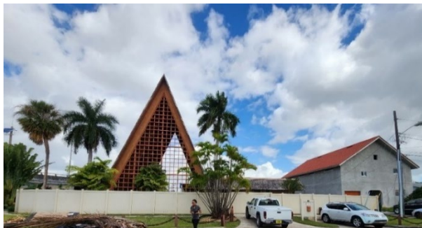
Subject property (left) and neighboring property, showing proximity and placement with land-side PVC property gate visible.
