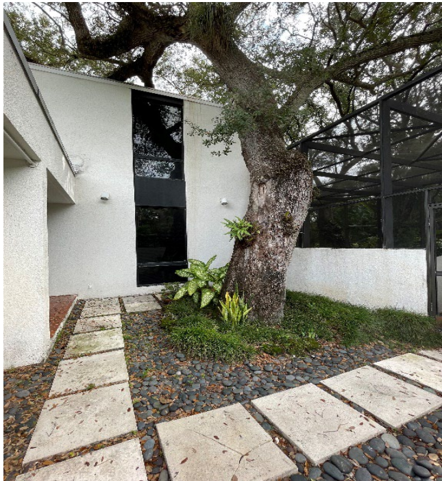
Courtyard at West façade 2024
