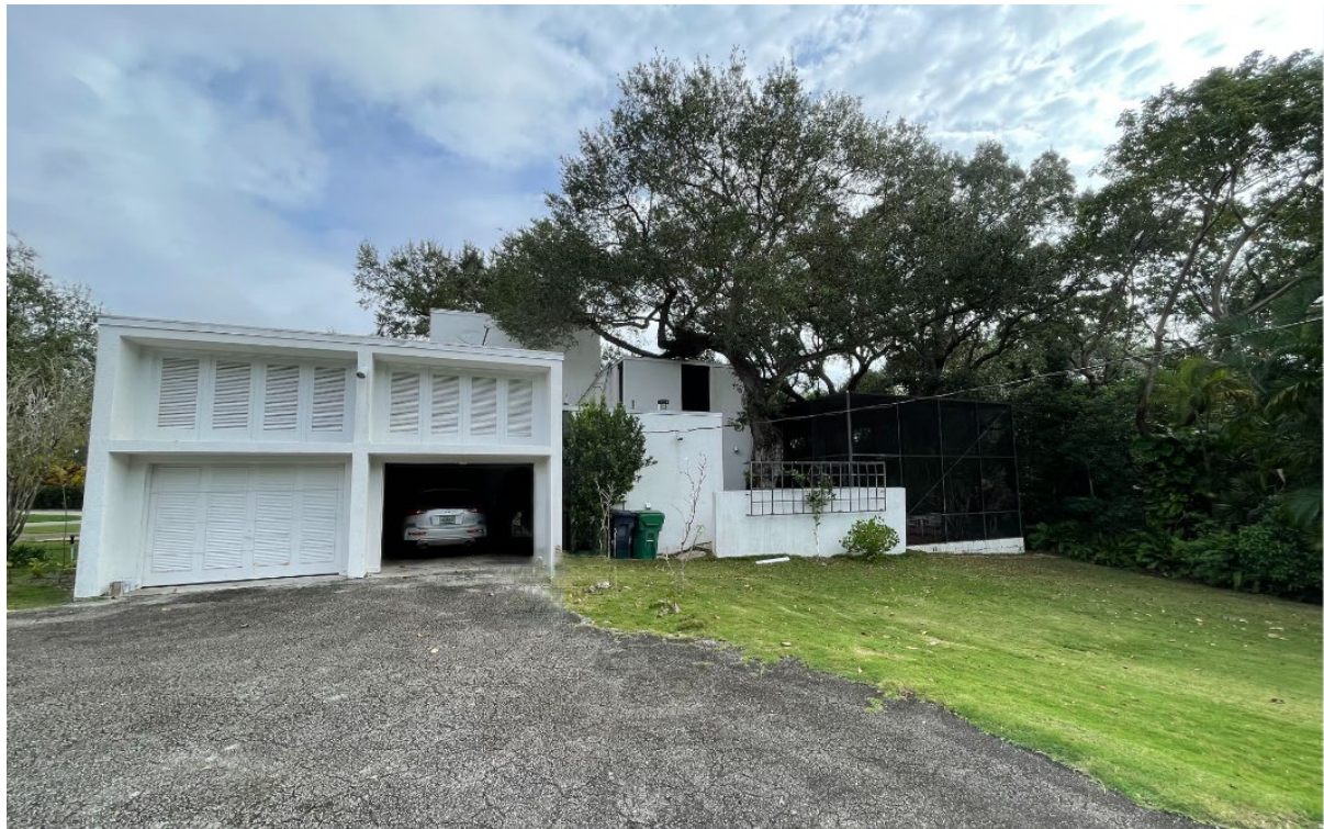
Garage at West façade with louvered doors 2024
