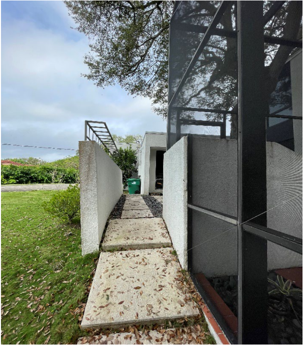
Courtyard privacy wall at West facade
