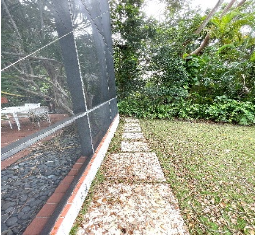
Sloped walkway at west façade
